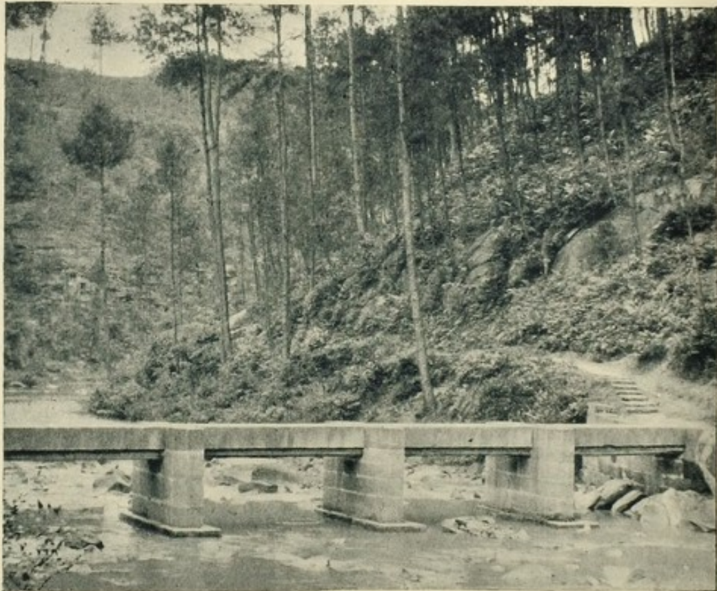
ONE OF CHINA'S BRIDGES.
