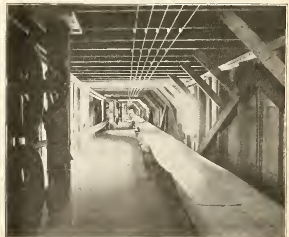
SINGLE BELT GALLERY AND ROPE TRANSMISSION.
