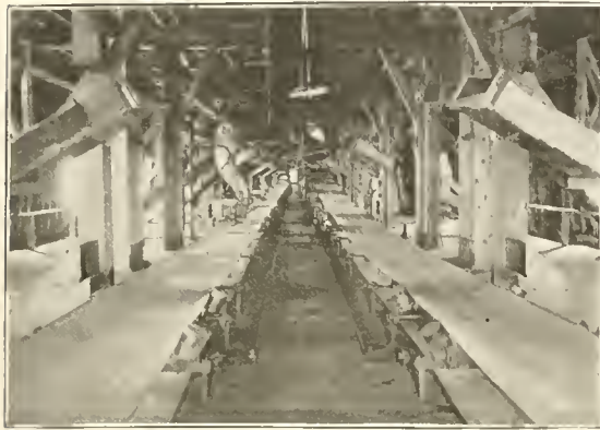
BELT CONVEYOR FLOOR.
