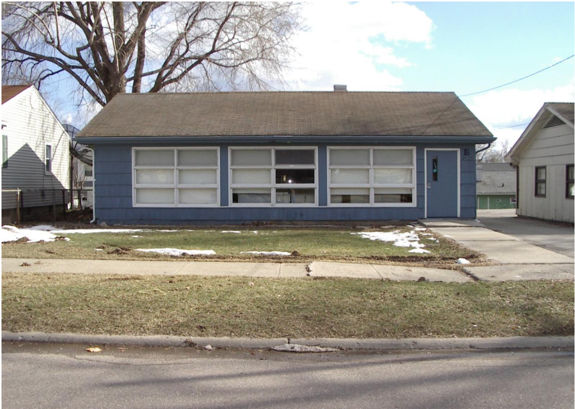
Figure 3.2. Primary unit. Once a primary unit for public school children, this structure on Flint’s west side now serves as a single-family home. Photograph by Andrew R. Highsmith, 2006.
