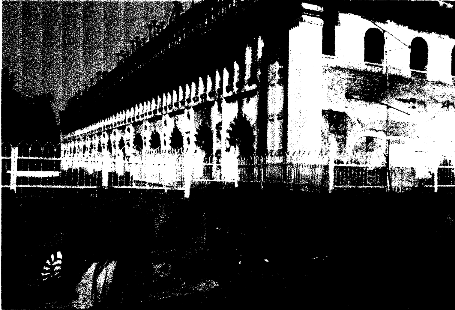
69. South exterior facade of Great Imbarah, photograph, March 2002
