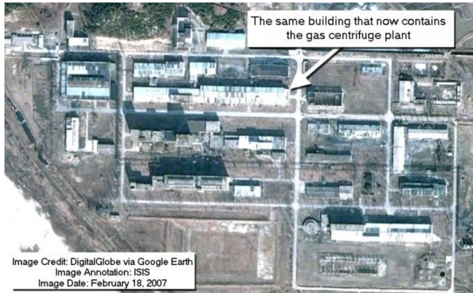
Figure 2: A view of the same building, then the fuel fabrication facility, that was later repurposed to make centrifuges (February 18, 2007).
