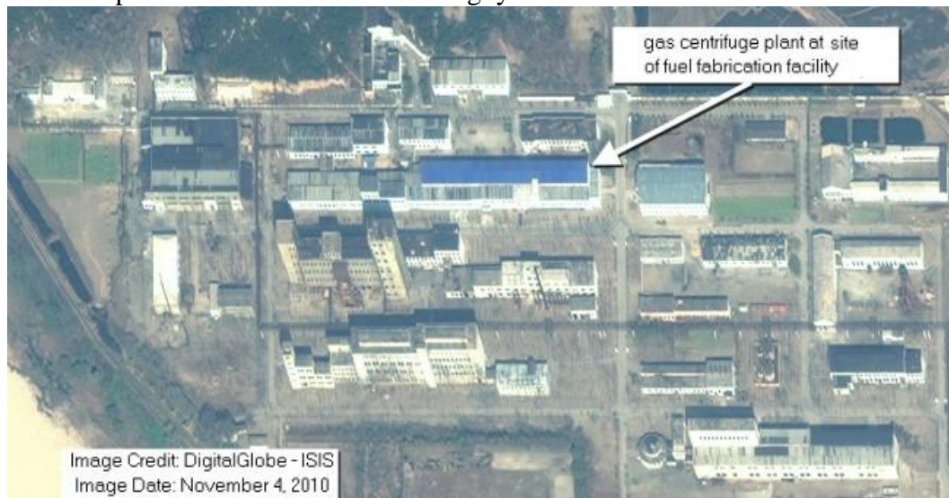
Figure 1: Satellite imagery of the North Korean uranium enrichment plant (November 4, 2010).
