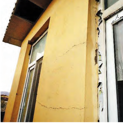
Construction deficiencies are already visible at a USAID-funded hospital in Gardez, Paktiya Province, completed in early 2016. (SIGAR photos)
