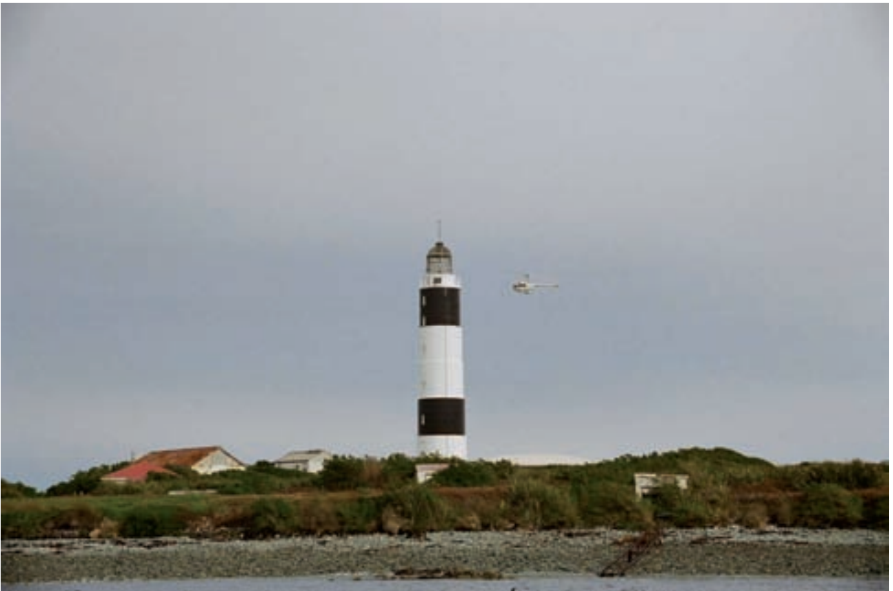
Dog Island lighthouse and cottages. Below the original cottage, 2008. R. EGERTON, DOC
