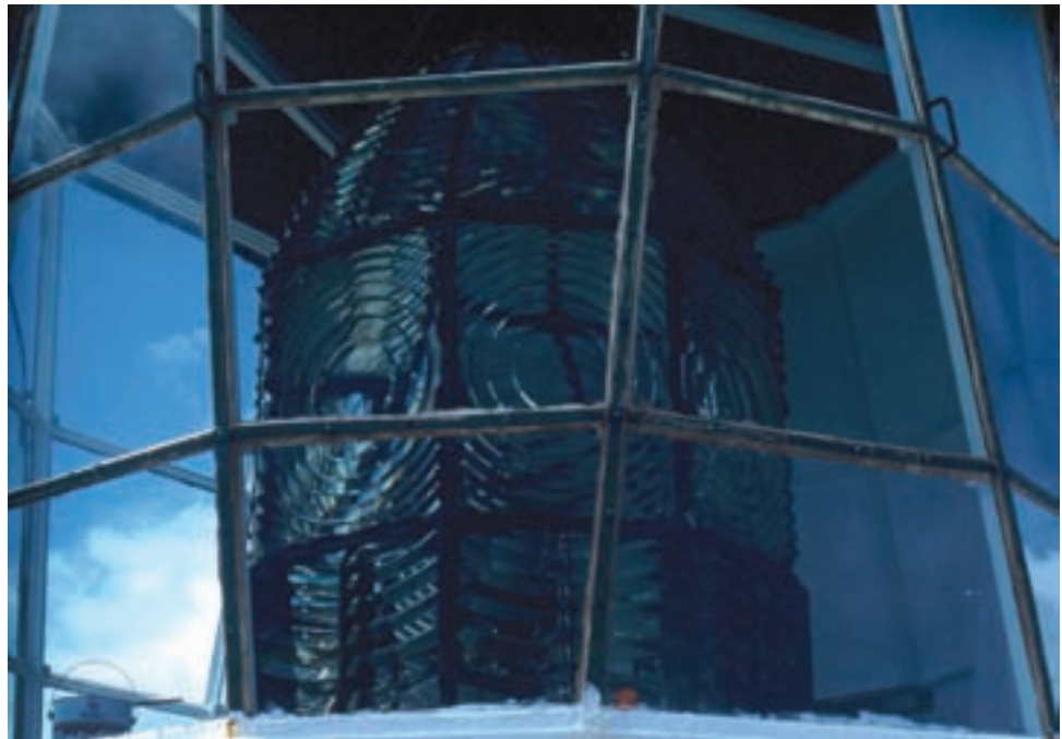
The automatic 'Austonlight' diesel-electric lighthouse system installed at Puysegur Point. DOC
