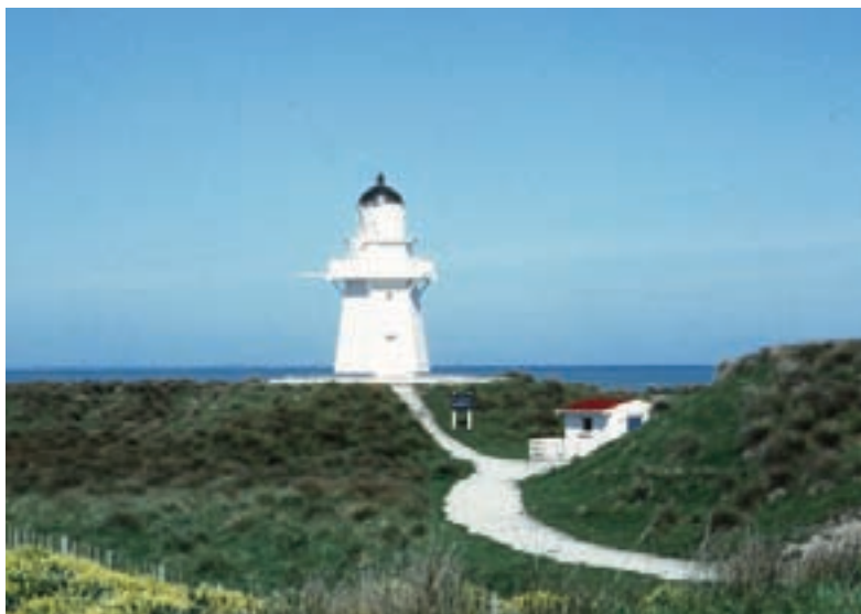
Waipapa & generator shed. COURTESY OF JANET RICHARDS
