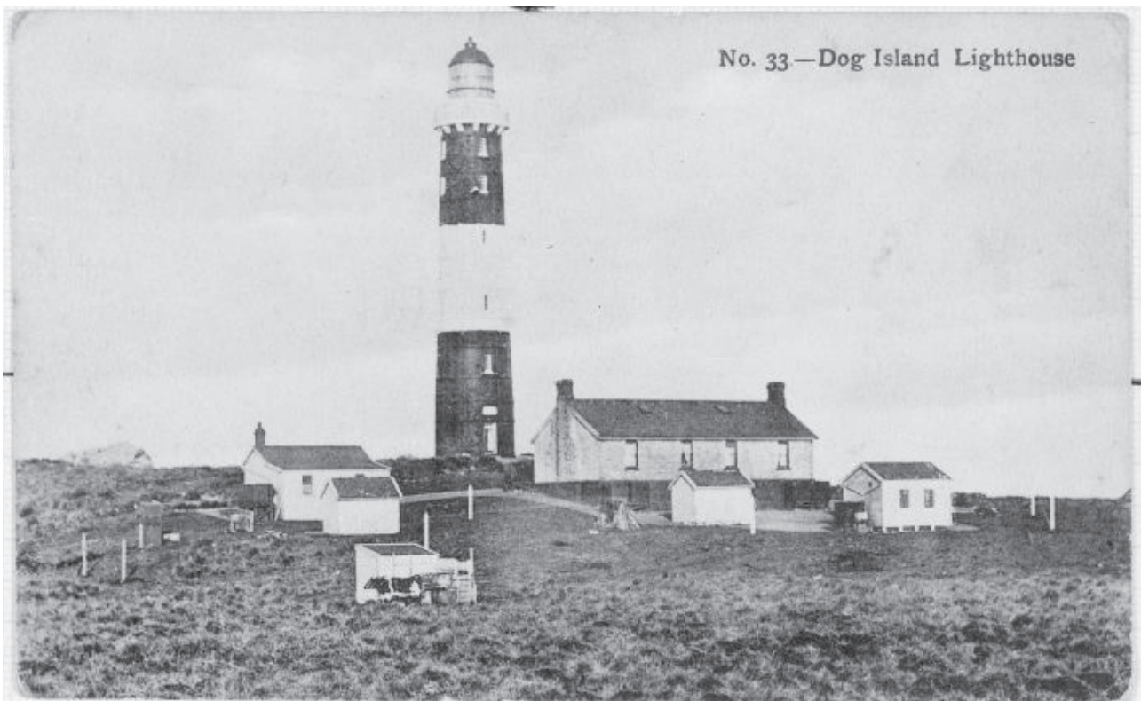
This photograph shows the 1863 building identified in the modern photograph. Dog Island Lighthouse. [190-?].
