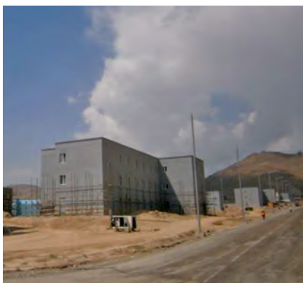
Afghan National Defense University , under construction, Kabul, September 2014. (USACE photo)
