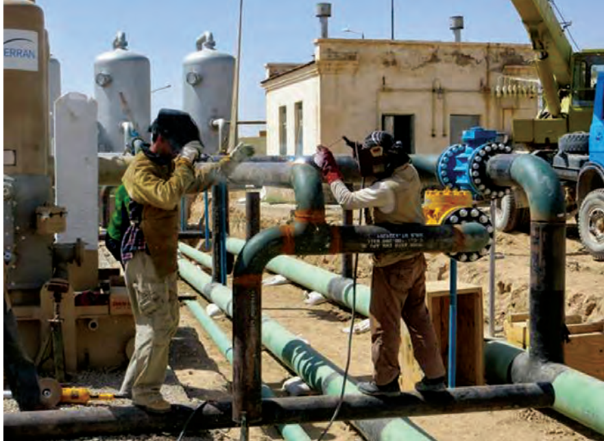
Workers weld a compressor pipe that is part of the Sheberghan pipeline-rehabilitation project. (TFBSO photo)
