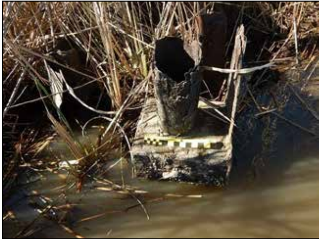
Figure 57. Probable bollard at southeast corner of Target 1, facing southwest.
