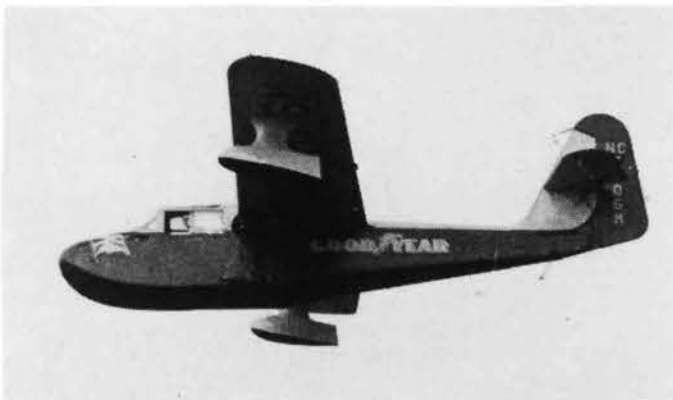
Above: NC5506M shows a clean profile with mainwheels and tailwheel retracted. (via Jack Meaden)
