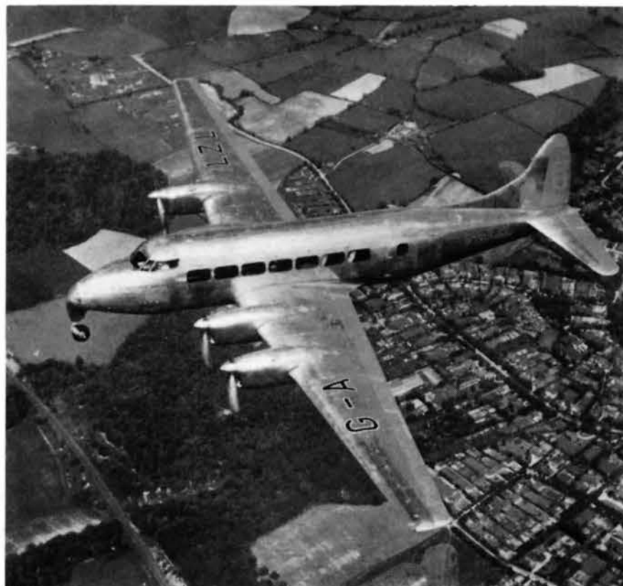
Above: Heron 1 prototype c/n 10903, built using Dove mainplanes, nose and tail but with a fixed undercarriage, photographed on an early flight.
