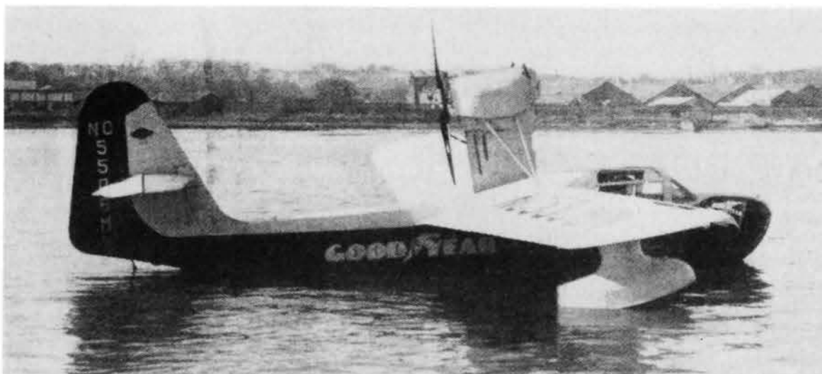
Above: NC5506M shows the low tail position of the GA-2 when in the water. (via Jack Meaden)
