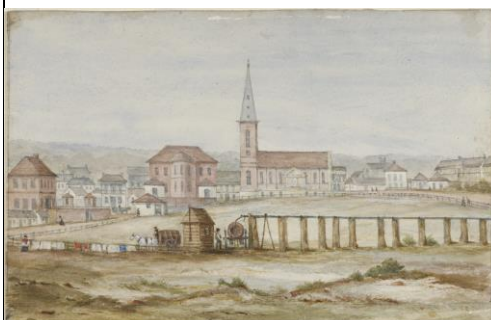
Busby's Bore piping at Hyde Park, n.d. (City of Sydney Archives)
