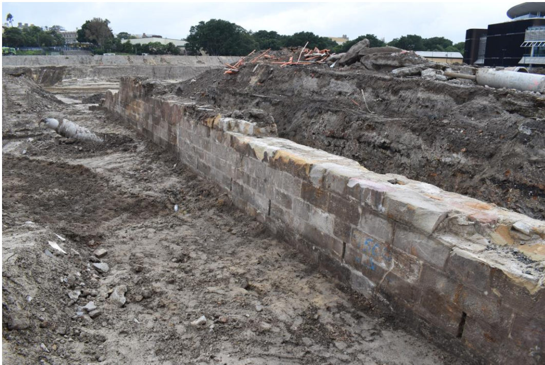
Figure 27. View of the large sandstone wall looking south-east.
