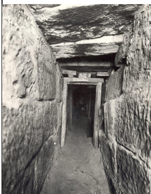
Busby's Bore under Oxford Street, Darlinghurst, constructed with stone masonry lining c.1820s-1830s (City of Sydney Archives)
