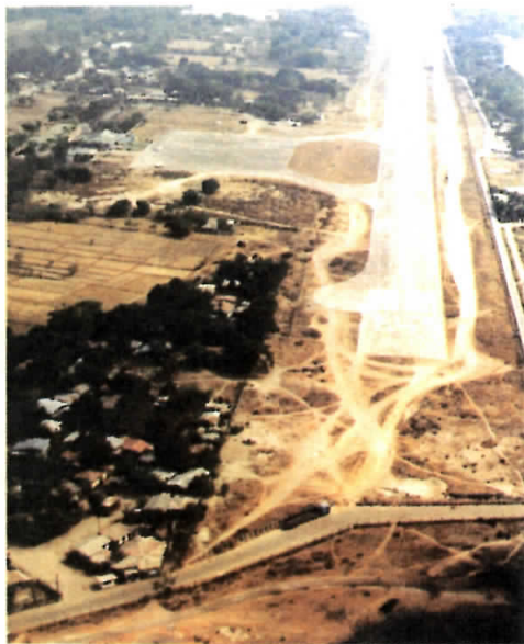
The San Fernando airport will be improved and its runway extended to accommodate Boeing 737 and Airbus 300 aircraft used in regional flights.
