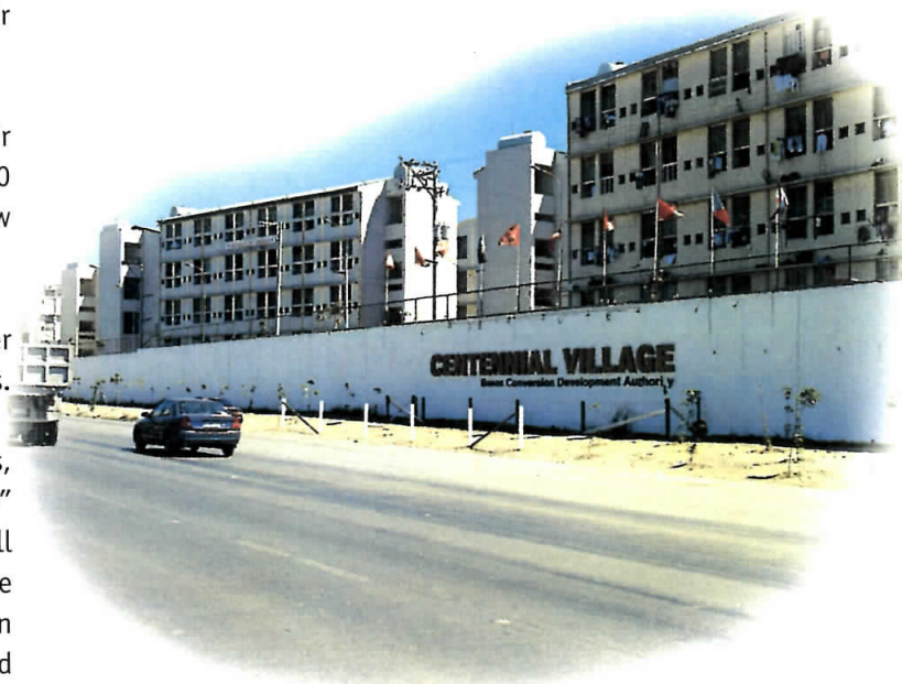
Centennial Village, one of BCDA's medium-rise projects and among the government's largest urban housing programs, is the home of some 741 military and civilian families.
