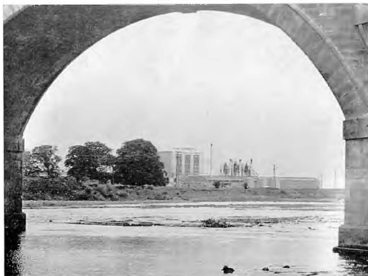
PLATE 36: The new chipboard factory at Hexham, Northumberland seen through the old bridge across the Tyne. This factory, though operating mainly on sawmill waste, is a potential user of thinnings from coniferous forests.
