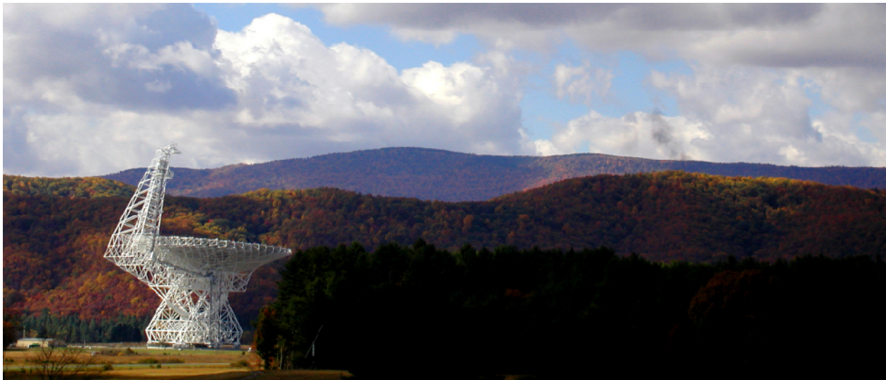
Figure 6.19. Robert C. Byrd Green Bank Telescope. This fully steerable radio telescope in West Virginia went into operation in August 2000. Its dish is about 100 meters across. (credit: "Cyberbaud"/Wikimedia)
