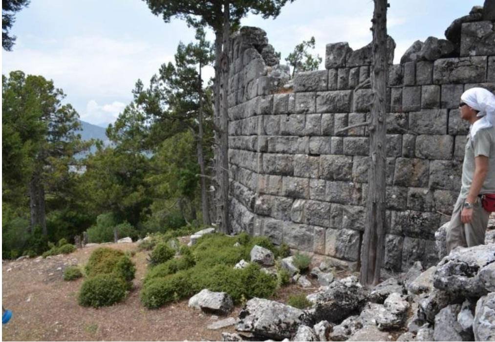
Figure 34. The Hellenistic isodomic, ashlar masonry of the pentagonal tower of Oinoanda. Taken by author in June 2015.
