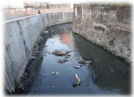
Station 5 (Las Piñas River) near CAA Bridge.
