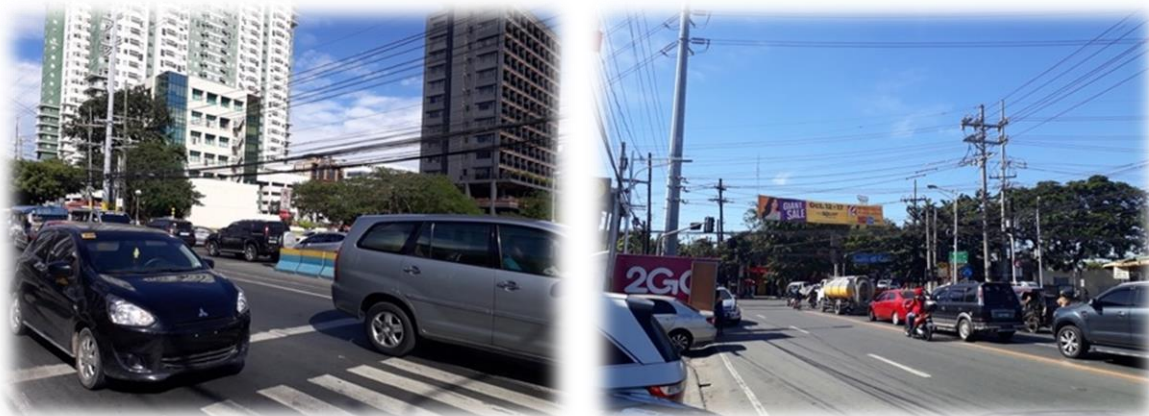
Plate 3-8. Sections of Alabang-Zapote Road in Muntinlupa City (left) and Las Piñas City (right).
