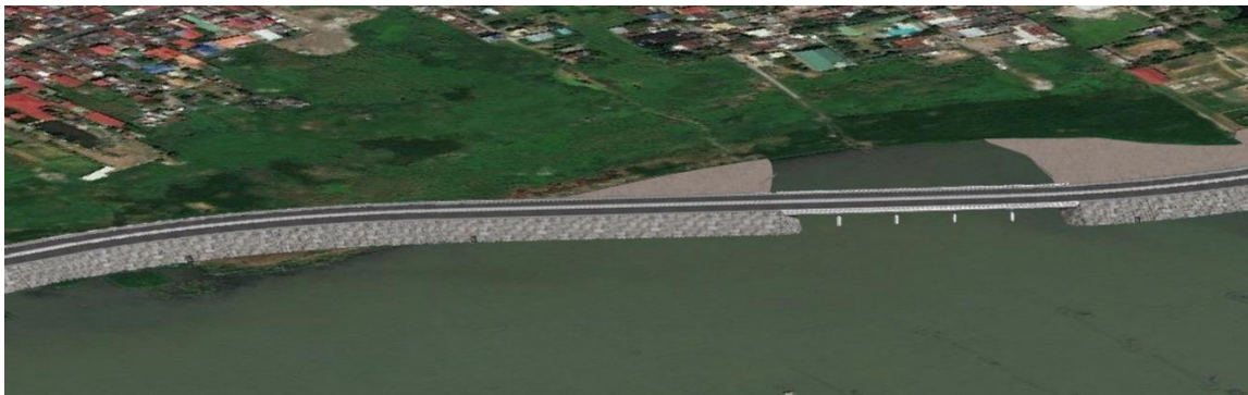
Figure 20 Embankment Viaduct at River outlet and fishery basin
