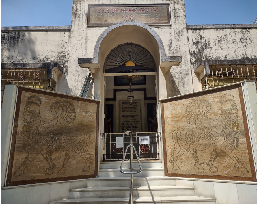
Fig. 2. Ustad Saheb Behramshah Nowroji Shroff Daremeher fire temple, Mumbai, India, 2023. Photograph © Mariano Errichiello.
