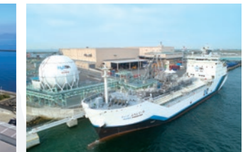
Liquefied hydrogen cargo handling demonstration terminal and liquefied hydrogen carrier, SUIISO FRONTIER
