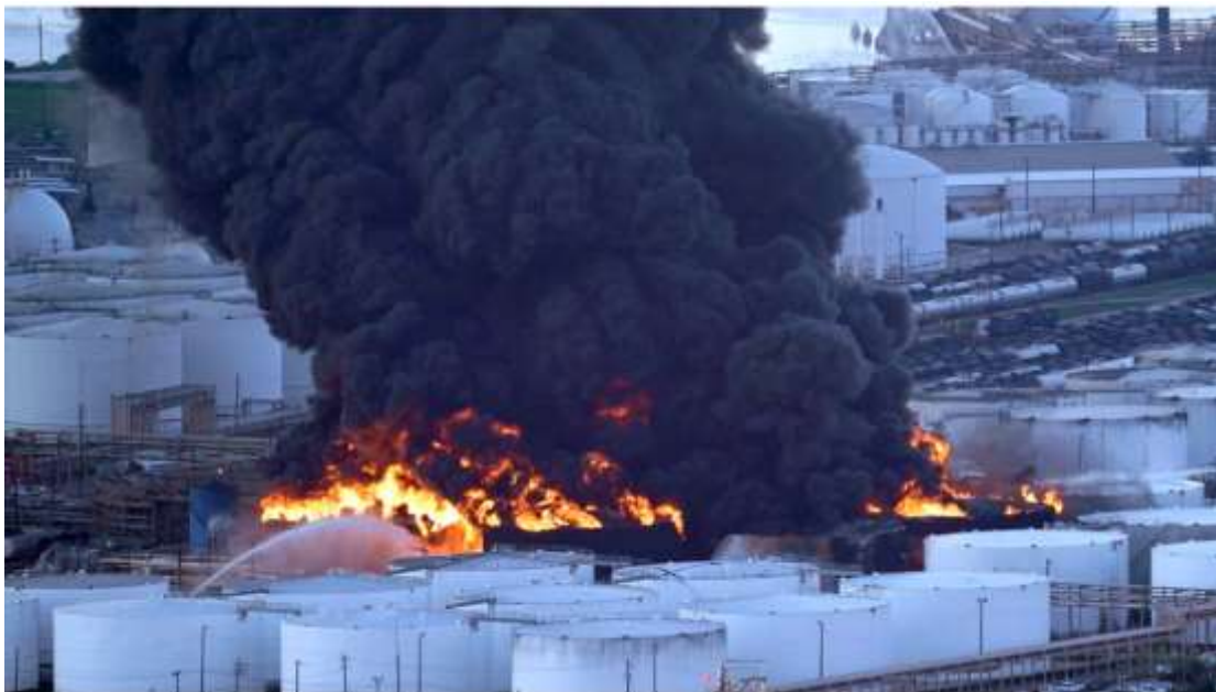
Fig. 2.2 Houston Tank Farm Fire Incident
