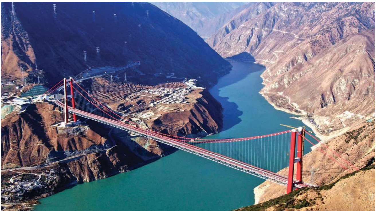
Figure 12.9: The Xingkang Jinsha River Bridge near Kangding on the G4218 YaYe Expressway
