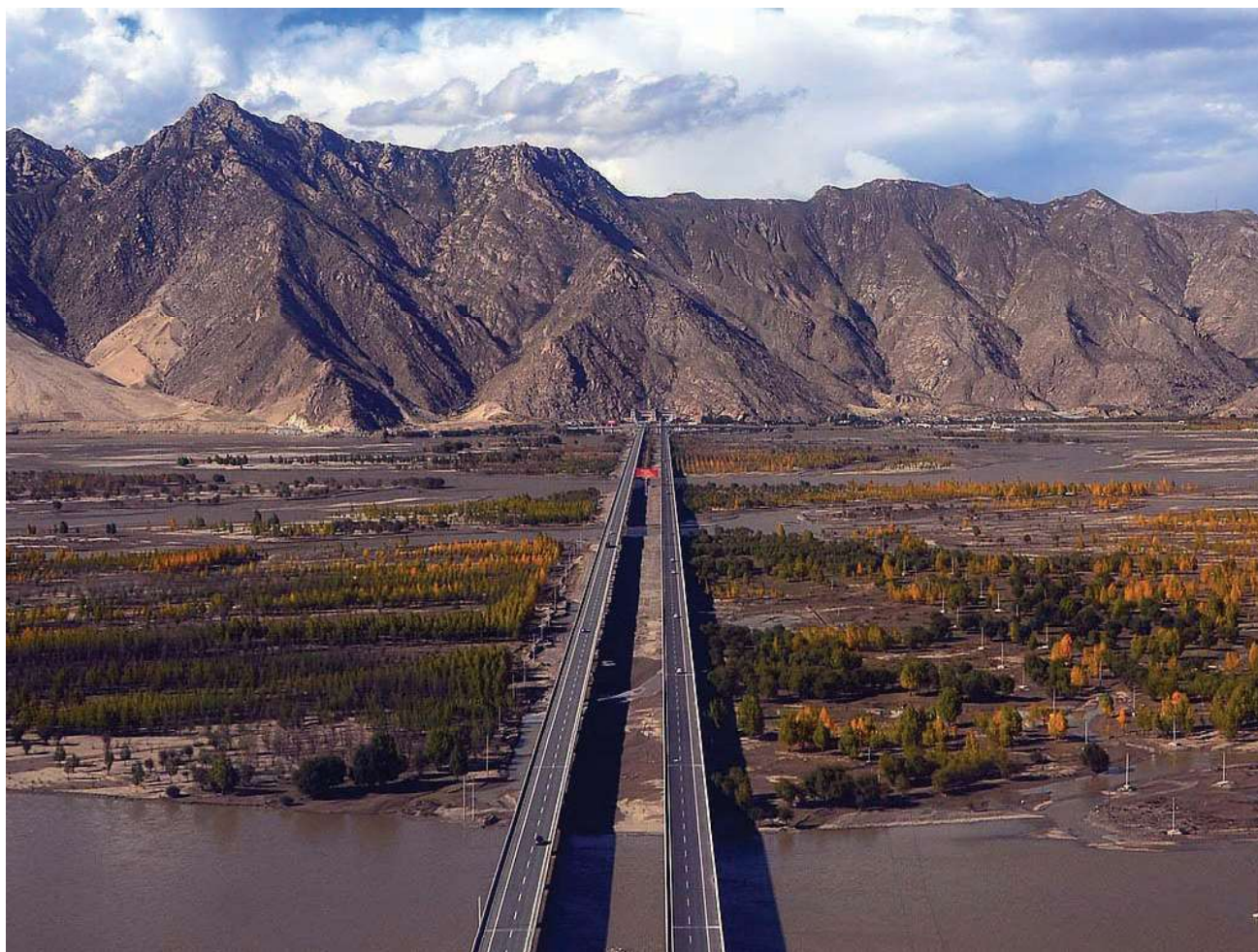
Figure 12.11: The Expressway to Lhasa Airport from Lhasa over the Yarlung Tsangpo River
