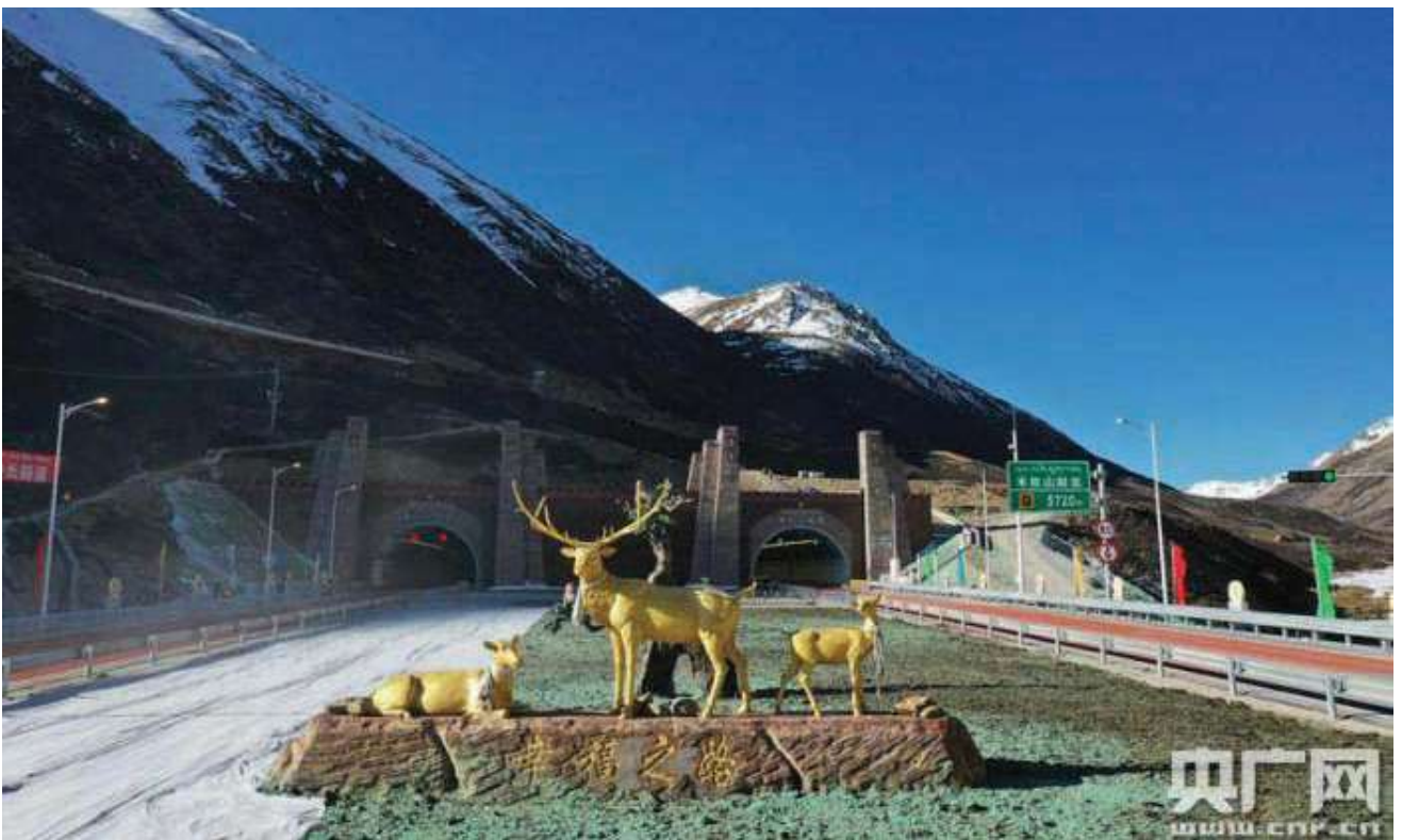
Figure 12.7: The World's highest tunnel, the Milashan Tunnel on the Lhasa Linzhi (Nyingchi) stretch of the G 4218 National Highway was opened for traffic on 26 Apr 2019. It is at an elevation of 4774 m. Each tube is 5727m and 5720m long.
