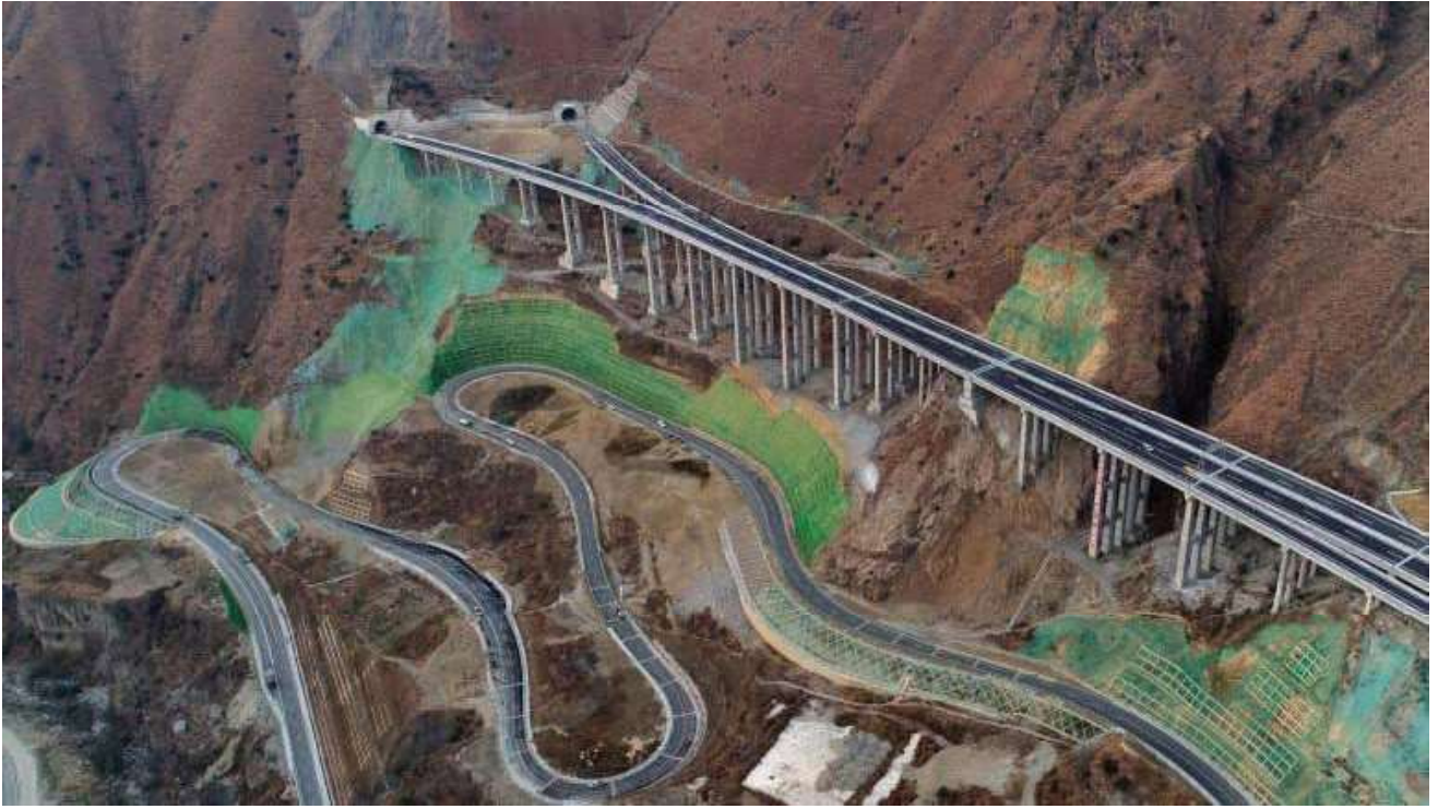
Figure 12.10: A view of the G4218 Yakang Expressway and the G318 Highway near Kangding. Copyright © 2017 CGTN
