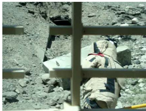
Figure A-5 EOD personnel in protective suit moves to inspect a culvert for an IED. Note the cement block dropped in front of the culvert as a barrier against robotic platforms.
