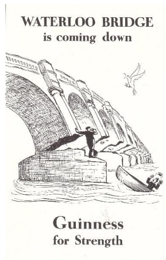
Figure 12. Waterloo Bridge demolition (1934) (Sibley 1985: 66).
