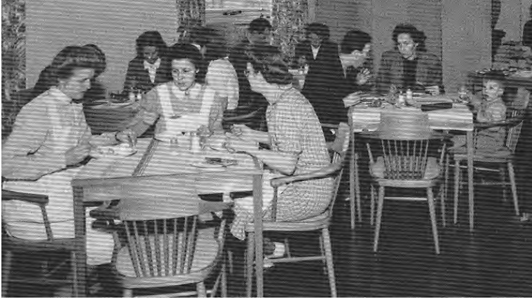
The dining hall of Marieberg collective housing. The tenants were required to buy 24 meal coupons per month. If they preferred, they could fetch a meal in a basket and eat in their apartments.
