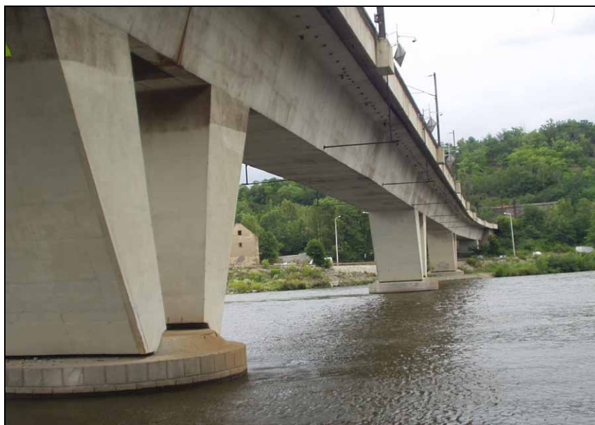
obr.3 TÚ: 0791 Praha Libeň – Praha Holešovice; km: 3,346
