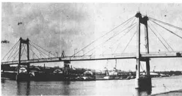
Figure 11. Dnieper Harbor Bridge.
