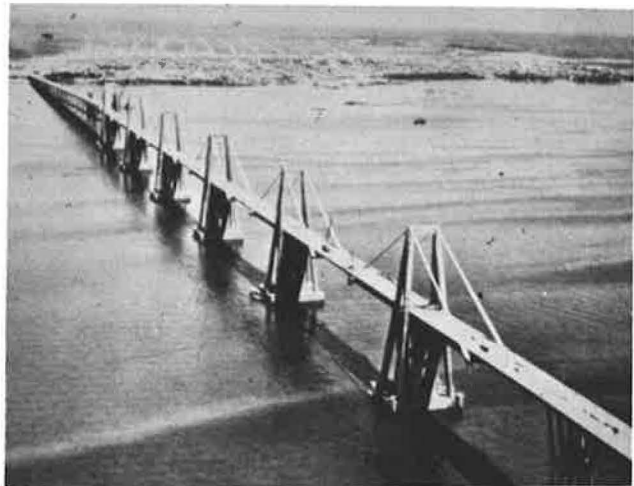
Figure 1. Lake Maracaibo Bridge.
