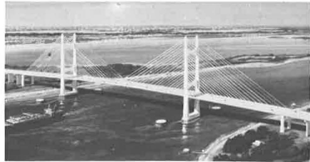
Figure 27. Dame Point Bridge.
