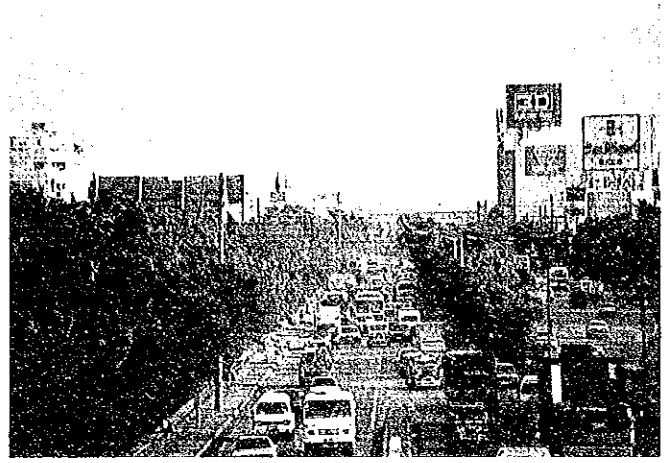
South Super Highway over which EXPRESSWAY ROUTE R-3 will be constructed.
