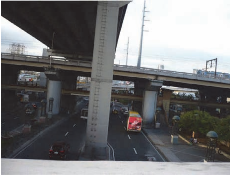
Photograph 5-4 Steel Pier and Steel Plate Girder
