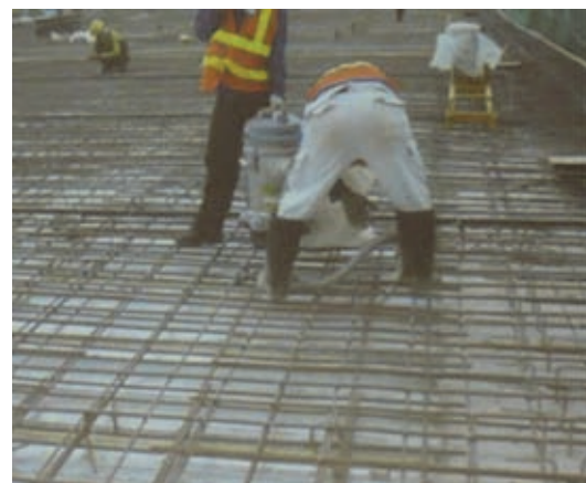
(b) Re-bars on Corrugated Steel Plate
