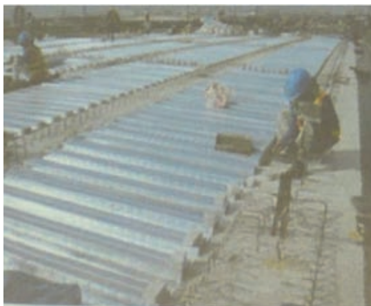
(a) Corrugated Steel Plate Work
