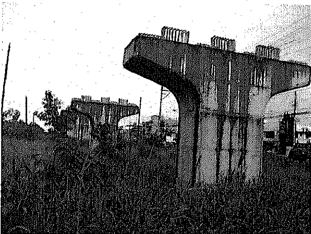
Figure 3.2-2 Uncompleted Substructure near Guiguinto and Substructure near Caloocan
