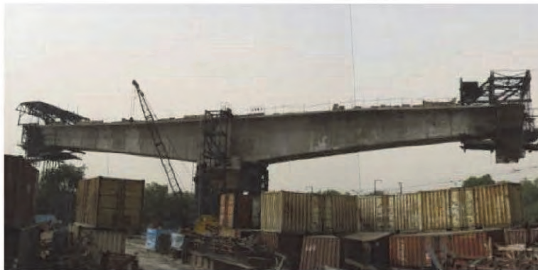
Figure 4.4.12 Long Span Bridge Delhi Metro Phase2, India
