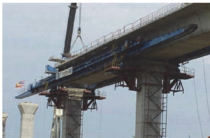
Figure 4.4.9 Example of Construction Method for Girder Erection
