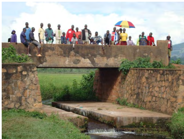
Wetland irrigation infrastructure rehabilitation is a popular intervention amongst international donors.
