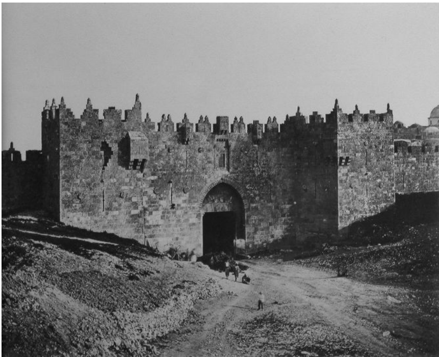
5. The Damascus gate in the walls of Jerusalem, these fortifications date from the Ottoman period.
