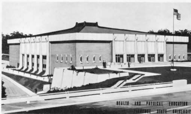
Florence State University's $3-million Health and Physical Education Building is now under construction and is expected to be completed by early 1972.
