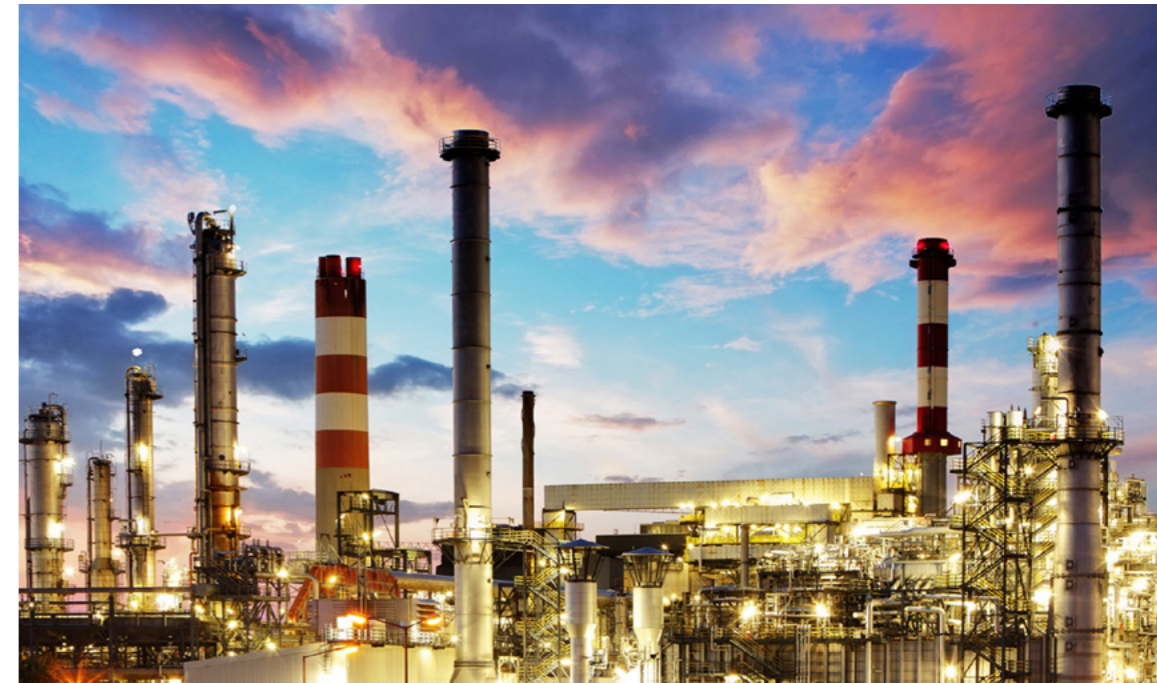
Dangote Refinery, Nigeria
