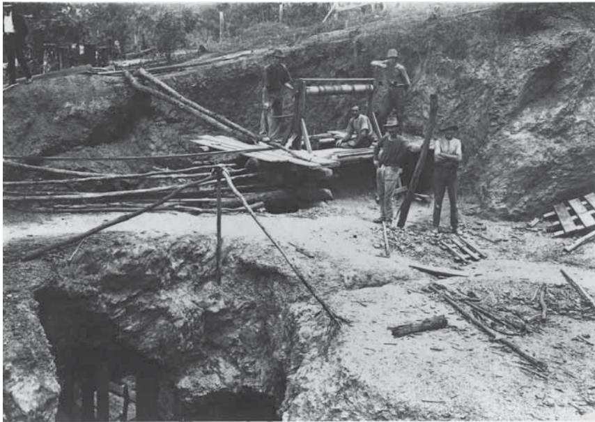
The rudimentary beginnings of Finney's Hill mine site
