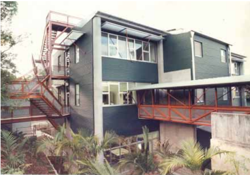
The finished Mineral Characterisation Research Facility
