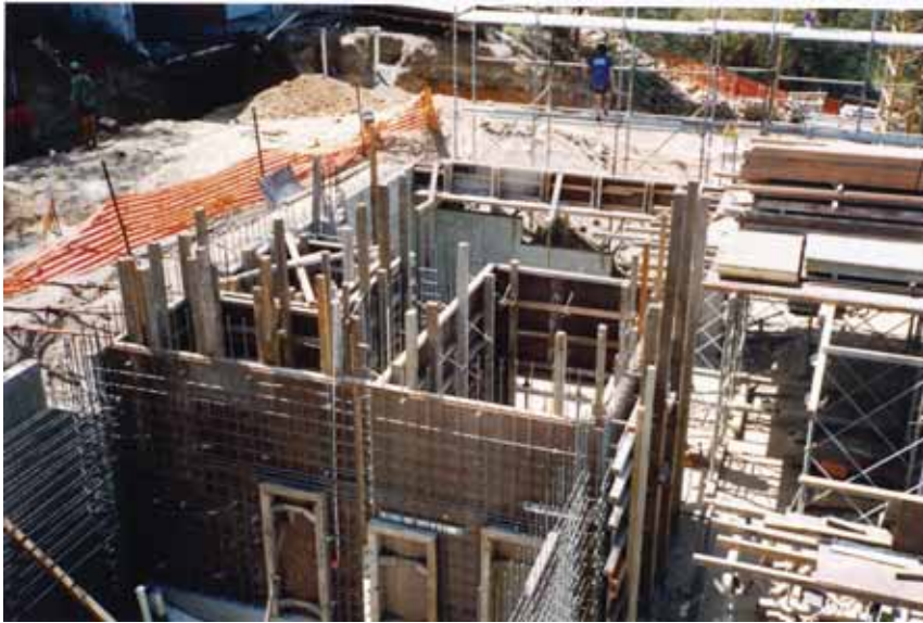
Preparation of Level 2 of the new Mineral Characterisation Research Facility
