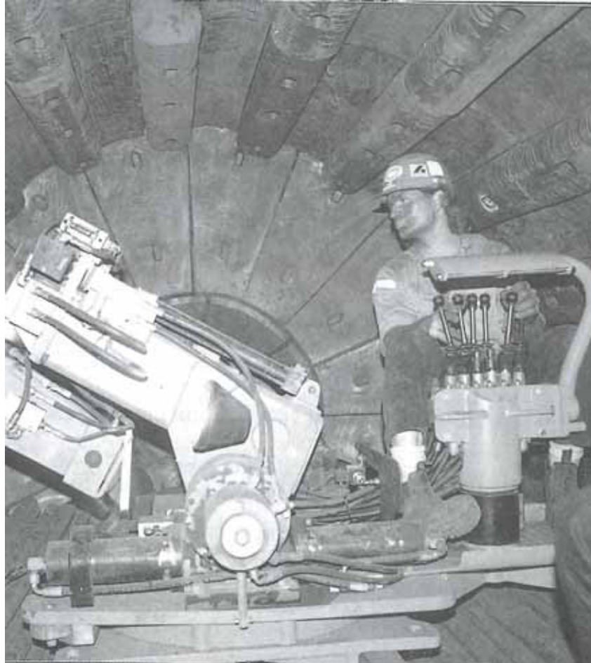
A mill relining machine operating inside a rod mill
