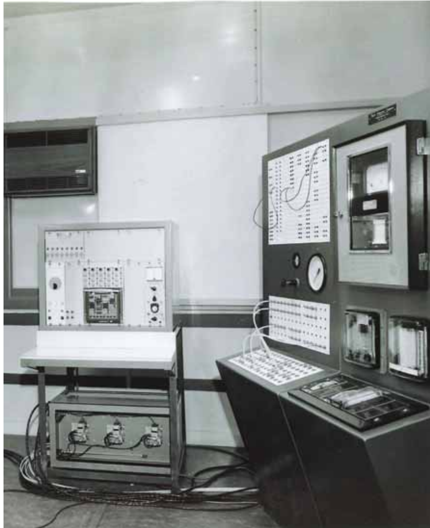
The former JKMRC Control Room
