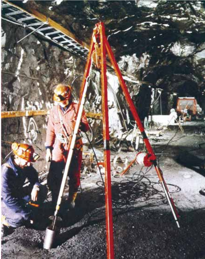
Undertaking a seismic scan in an underground tunnel
