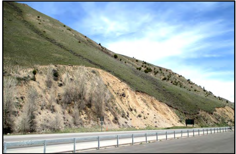
Figure 3: East slope of East Gros Ventre Butte just north of the Jackson town line along Highway 89 showing a typical slope and removal of buttress material to build the highway.
