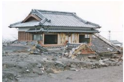
Figure 1: Building destroyed by eruptions at Mount Unzen, Japan
