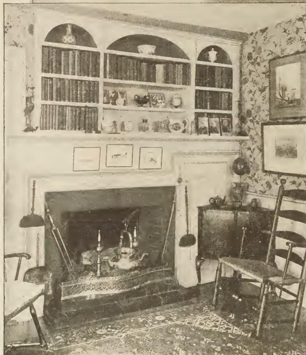
AT FIRST THE FIREPLACE SMOKED A GOOD DEAL, BUT TWO LAYERS OF BRICK LIFTED THE HEARTH ABOVE THE FLOOR-LEVEL AND STOPPED THIS NUISANCE
