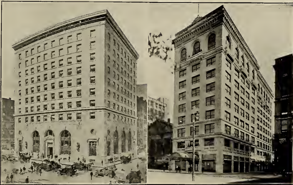
Boston Safe Deposit Bldg.
