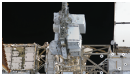
Exterior nadir view of the EXPRESS Logistics Carrier 1 (ELC1) mounted to the P3 truss segment.
