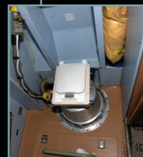
Toilet Compartment in the Service Module (SM) / Zvezda.
