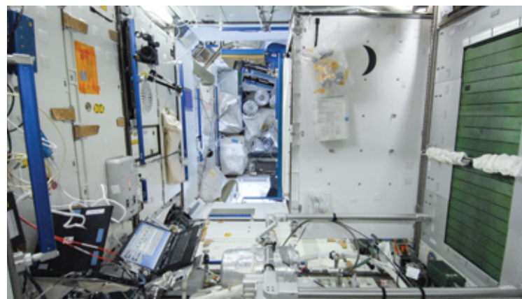
View of the Waste Management Compartment (WMC) in the Node 3 module.
