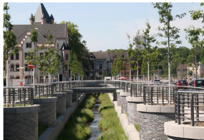
Urban integration of natural River Emscher at Lake Phoenix (Photo by Wirtschaftsfoerderung Dortmund)
