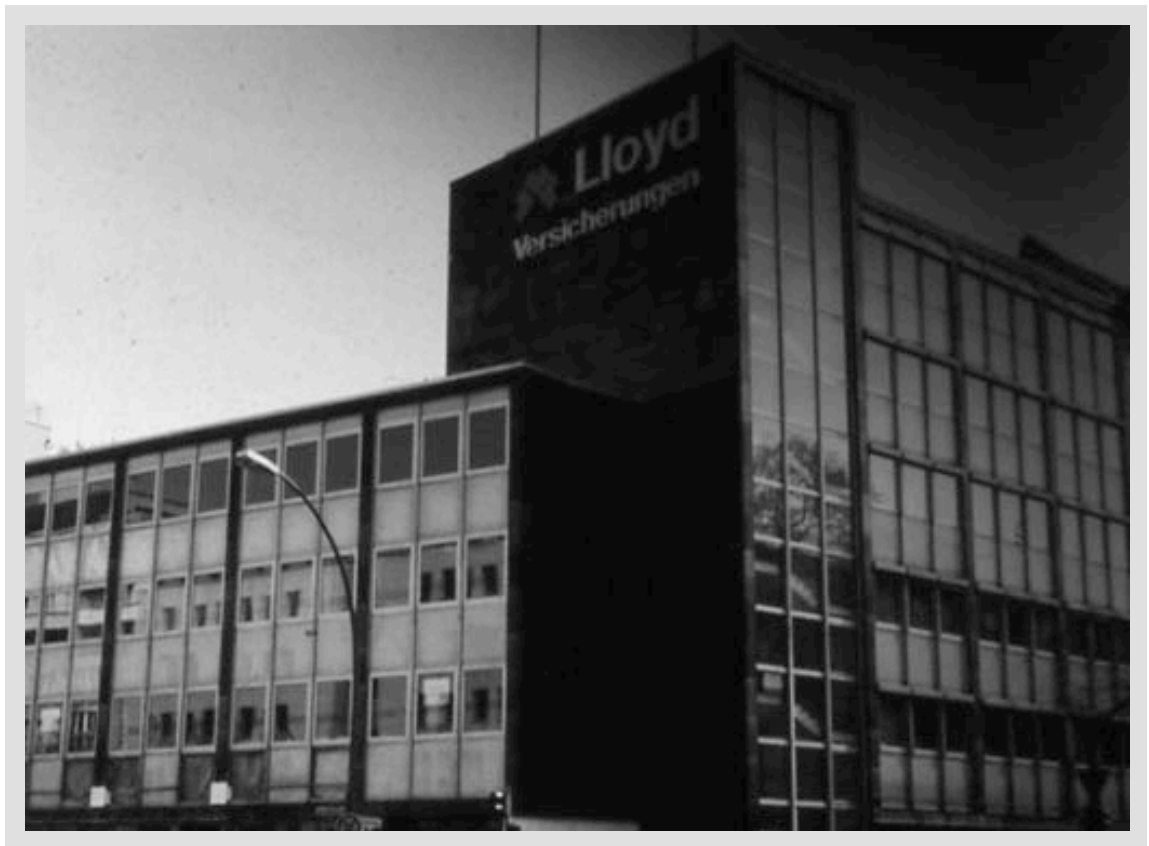
Illustration 7 | 34 Sigrid Kressmann-Zschach, Lloyd Insurance Building, Uhlandstraße 75 West Berlin, 1955
