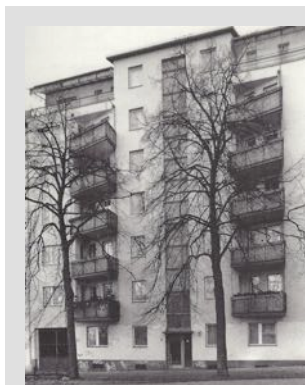
Illustration 7 | 19 Hilde Weström, residential building, street view, Mecklenburgische Straße 86, West Berlin, 1955
