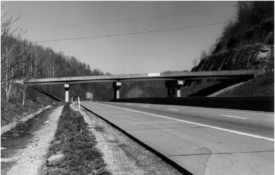
Exhibit 10-4. Typical Grade Separation Structure With Open-End Span
