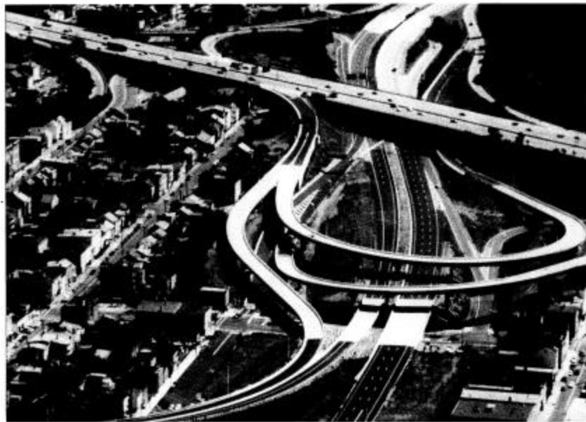
Exhibit 10-41. Complex Interchange Arrangement
