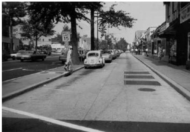
Exhibit 4-12. Frontage Road in Business Area With Narrow Outer Separation
