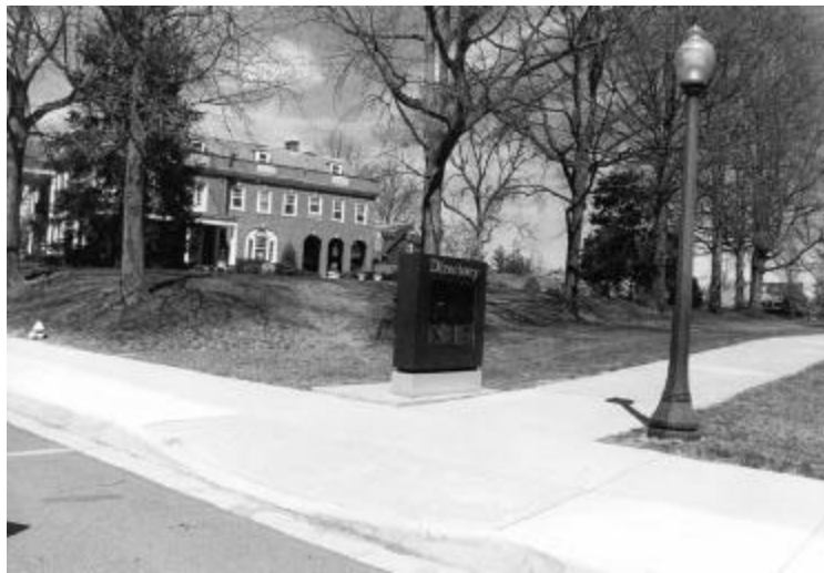
Exhibit 4-25. Sidewalk Curb Ramp at Midblock
