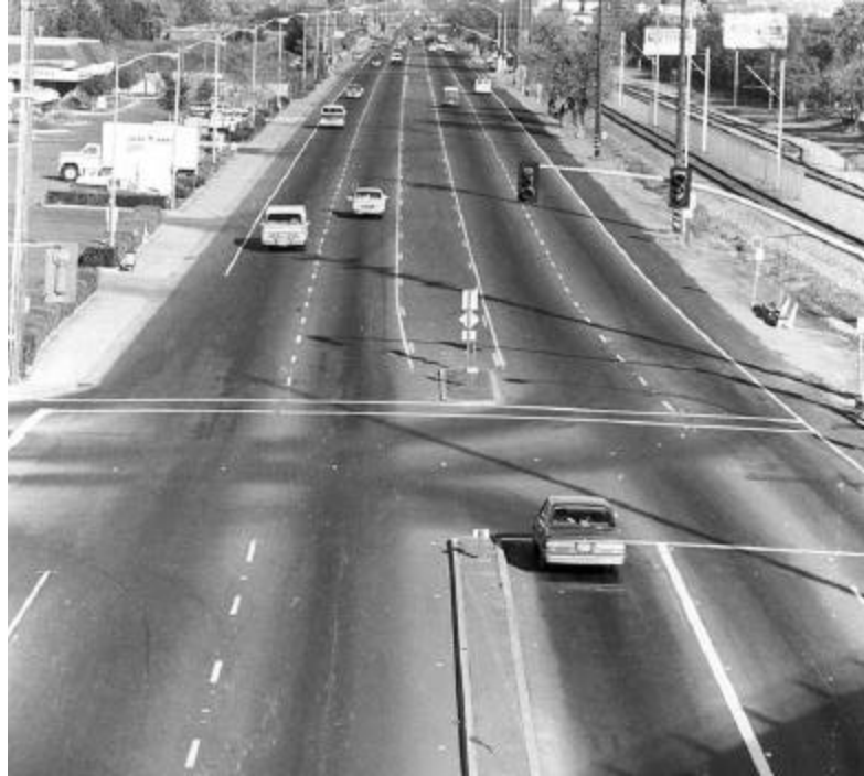
Exhibit 7-11. Continuous Two-Way Left-Turn Lane
