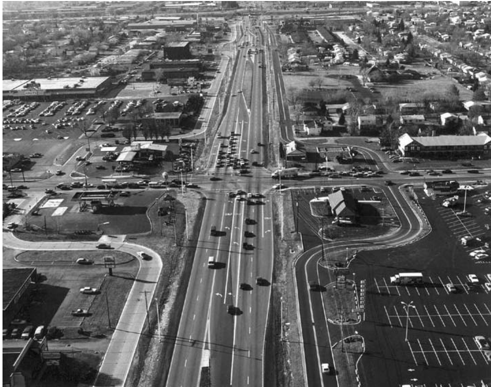
Exhibit 7-16. Divided Arterial Street With Two-Way Frontage Road
