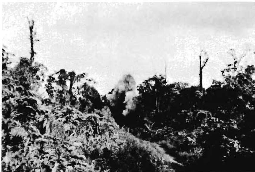
Figure 104. Solid pahoehoe outcropping at Keaau Orchard being blasted with dynamite charges to establish orchard at Keaau, Hawaii, December 1949. (Courtesy of Mauna Loa Macadamia Nut Corp.)
