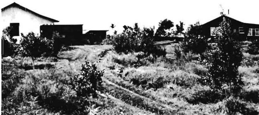
Figure 94. The Keauhou warehouse in Kona, built in the early 1930s, was already in bad condition when the authors saw it in the early 1950s.
