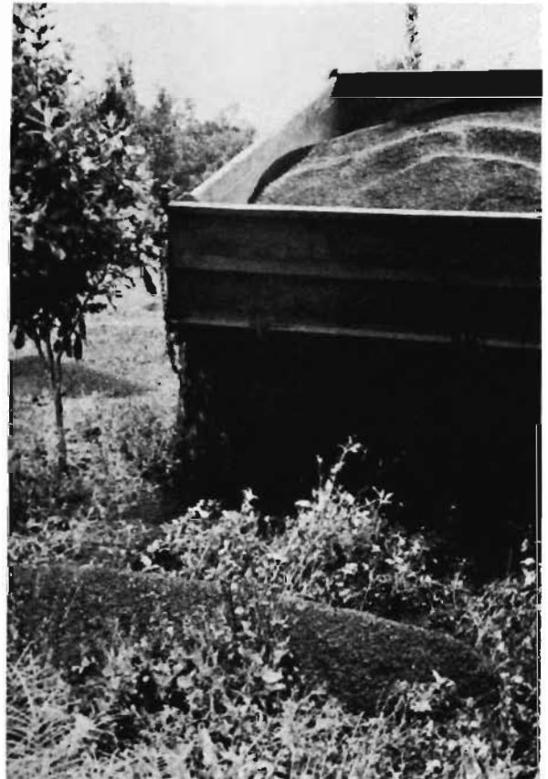
Figure 107. The use of fines and waste from the quarry in Hilo to give lava land a smooth finish without any deep crevices, 1950. (Courtesy of Mauna Loa Macadamia Nut Corp.)
