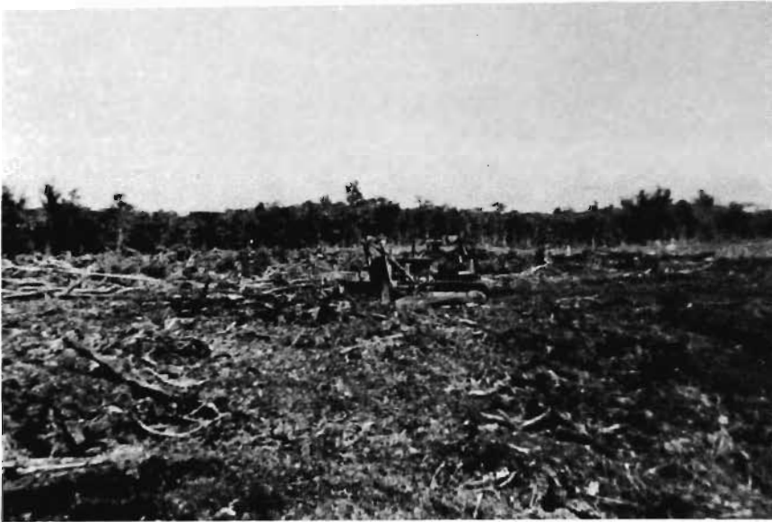
Figure 105. Leveling cleared land and pushing vegetation into huge piles to burn at Keaau Orchard, 1949. (Courtesy of Mauna Loa Macadamia Nut Corp.)
