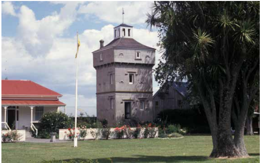
Figure 40. Firth's Tower, Matamata: built 1881–82 as a look-out and refuge on J.C. Firth's 23,000 ha Matamata Estate. Photo: N. Prickett, 2001.
