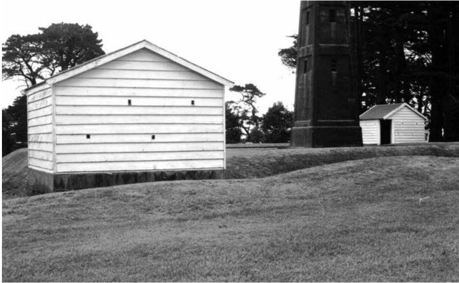
Figure 105. Manaia Redoubt: the Parihaka Campaign fortification has two blockhouses at opposite angles for flanking defence. A concrete tower at the centre of the square redoubt replaces the original wooden watch-tower. Photo: N. Prickett, 1975.
