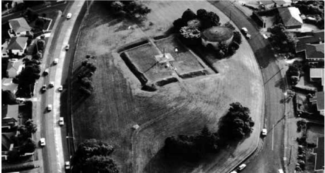
Figure 21. Howick Stockade; the defensive ditch outside the stockade defence has been subject to reconstruction. Photo: N. Prickett, 1992.
