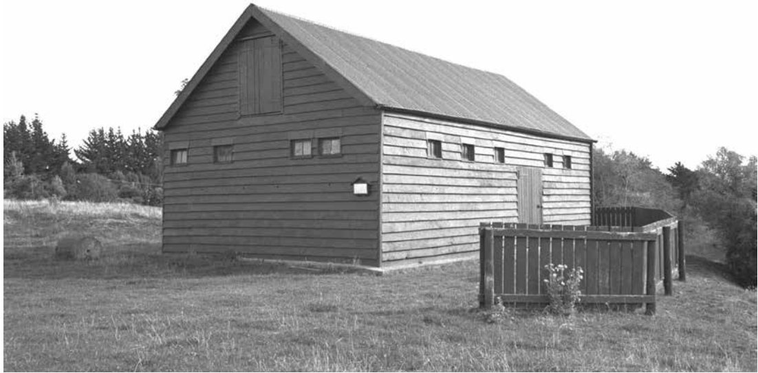
Figure 8. Marangai Blockhouse (1.50), Whanganui: example of single-storey fortification; restored in recent years, with added concrete base. Photo: N. Prickett, 2001.
