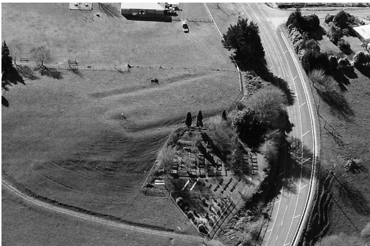
Figure 41. Ohaupo Redoubt, from the south, Ohaupo Road (SH3) at right. Photo: K.L. Jones, 2004.
