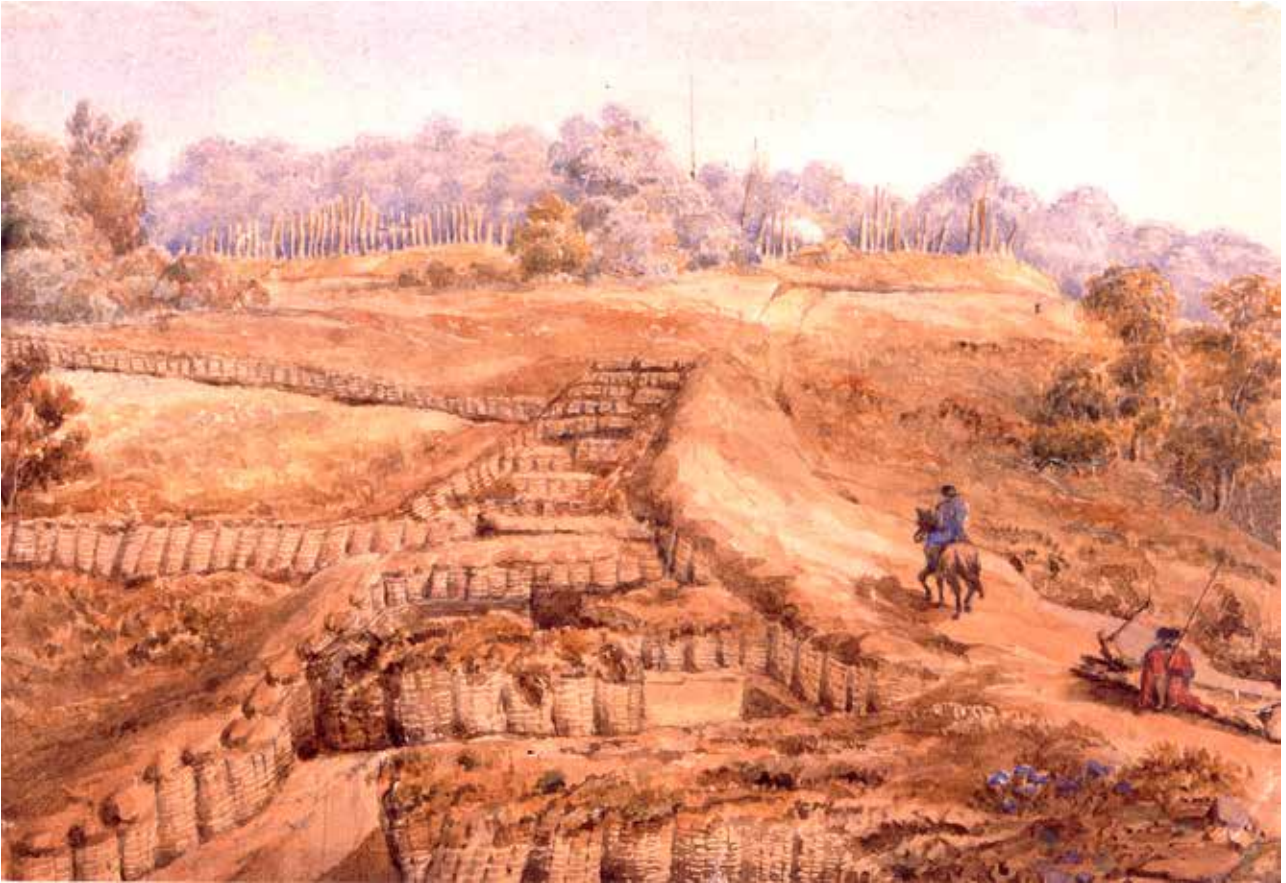
Figure 86. 'The Limit of the Sap at Te Arei', 1861. Picture immediately after the March 1861 ceasefire shows the use of traverses and wicker gabions to prevent an enfilading fire. At left are two demi-parallels extending to the cliff to the river; beyond is Te Arei pā. Francis Hamar Arden, watercolour, collection of Puke Ariki, New Plymouth, (A75.439).
