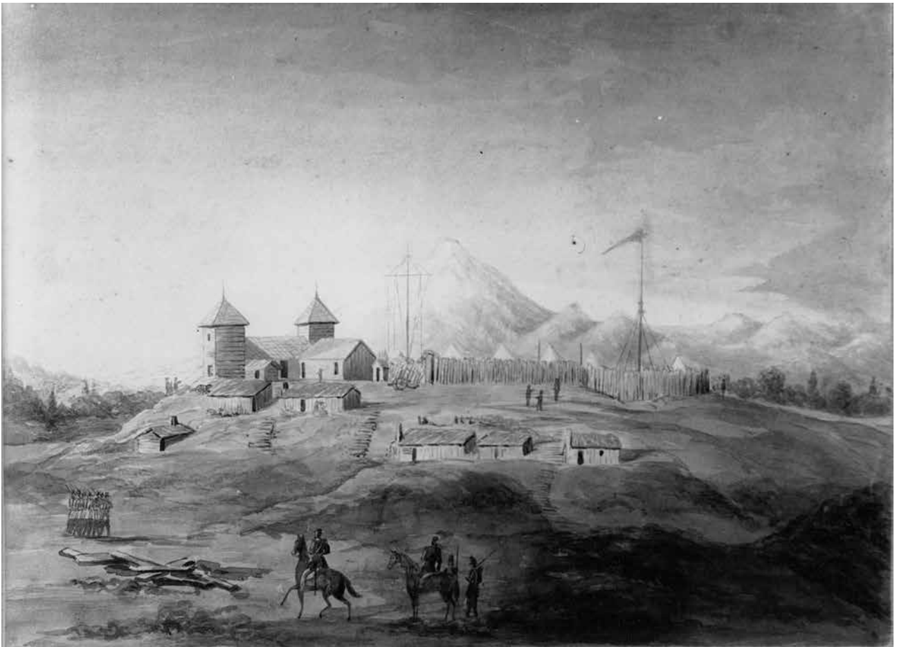
Figure 71. 'Bell Block Stockade'. View from the northeast, at left is the blockhouse with two bastion towers and to the right is the added stockade. Francis Hamar Arden, pencil and wash, collection of Puke Ariki, New Plymouth, A75.453.
