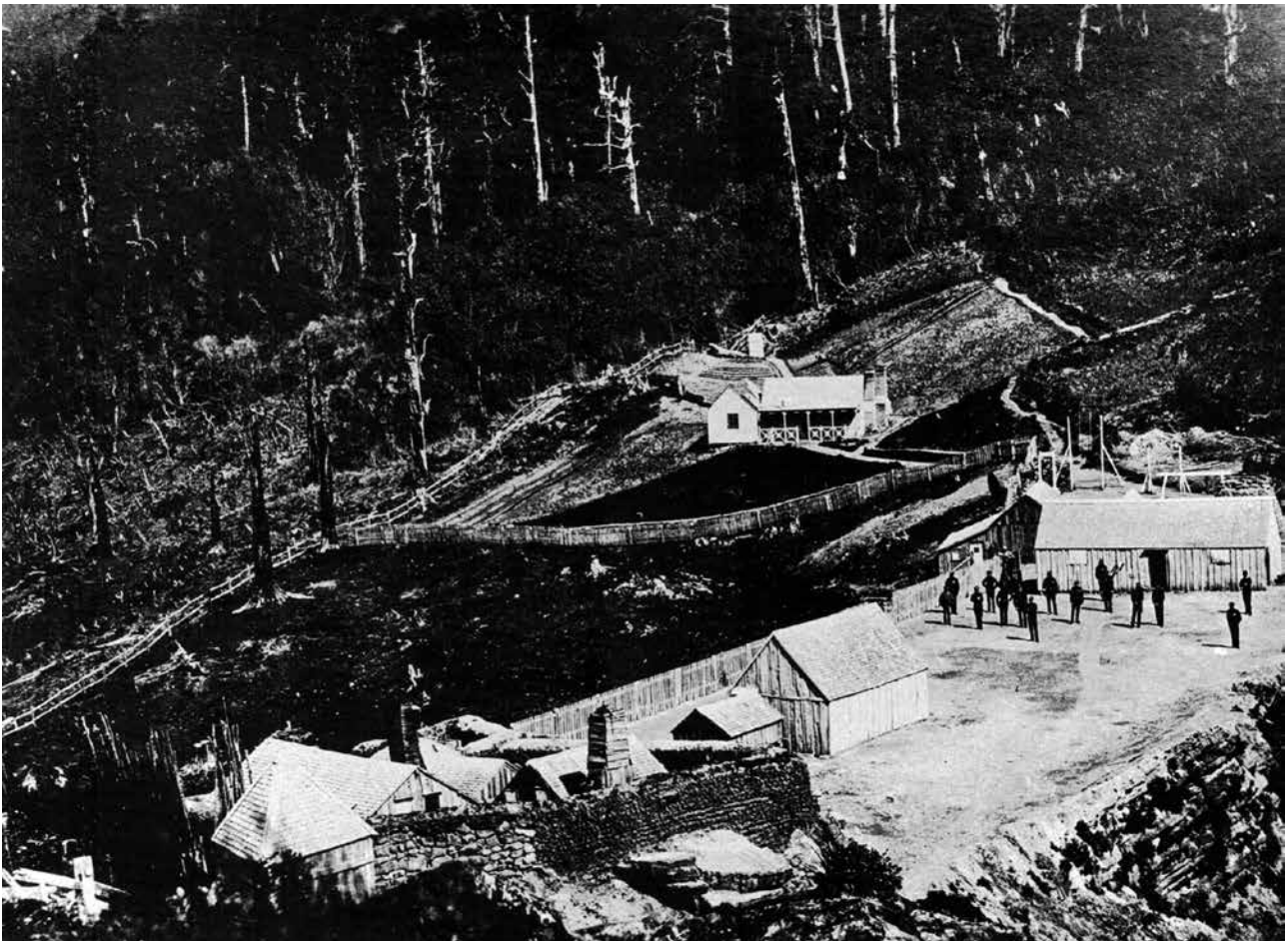
Figure 67. Onepoto Redoubt, Lake Waikaremoana: buildings fill the interior of a small redoubt of earth and stone walls. Photographer not known, Ref: 1/2-020463-F, Alexander Turnbull Library, Wellington.
