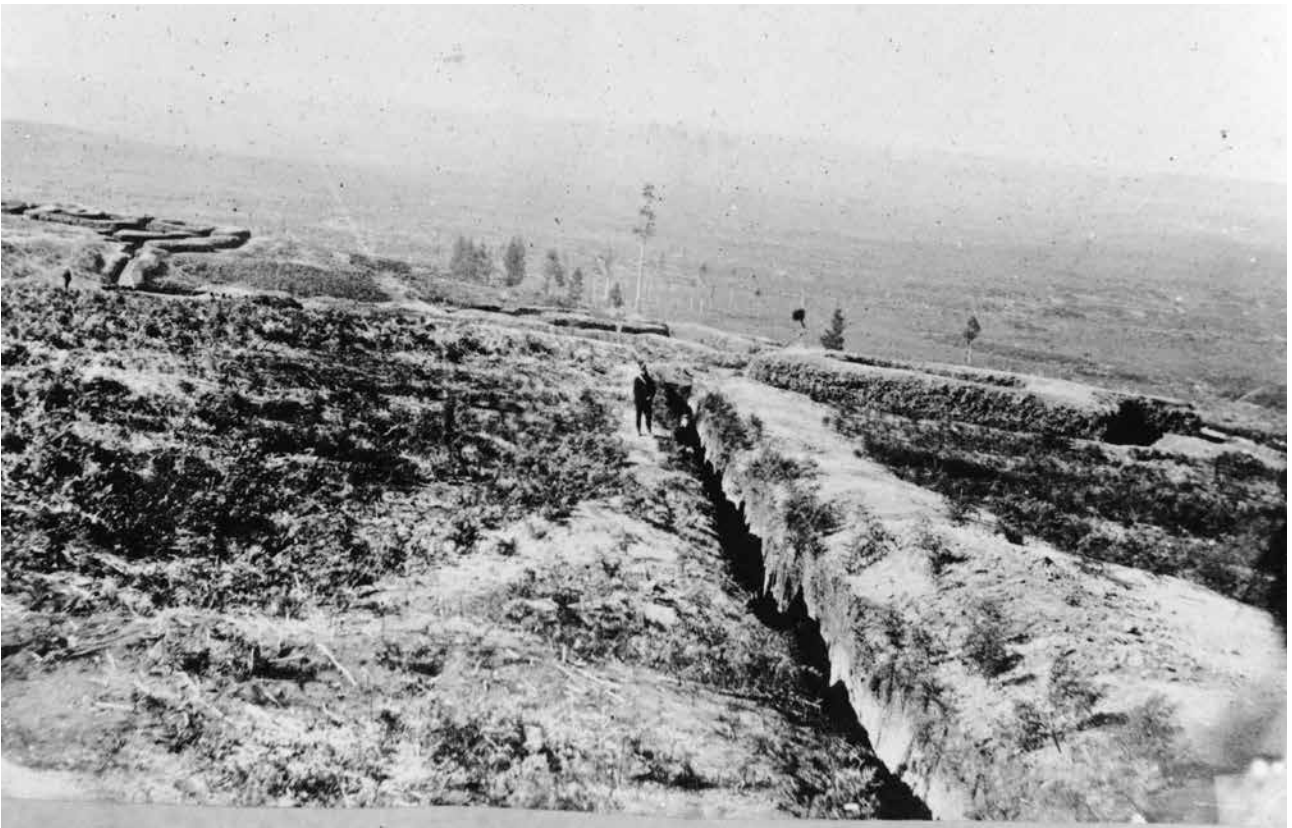
Figure 37. Paterangi: the largest continuous barrier pā of the New Zealand Wars included nine strong points, two of them shown here at right and left distance, with rifle trenches between. Photo: M. Higginson (attributed), Auckland Museum album 510, p. 6.
