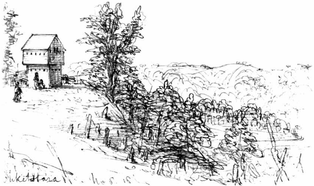
Figure 9. 'Puketotara Nov. 18' [1864]. Puketotara Blockhouse (9.22), near New Plymouth, is an example of a two-storey work. Colonel H.J. Warre, Sketchbook 1864-1865, p. 51, Ref: E-294-051, Alexander Turnbull Library, Wellington.
