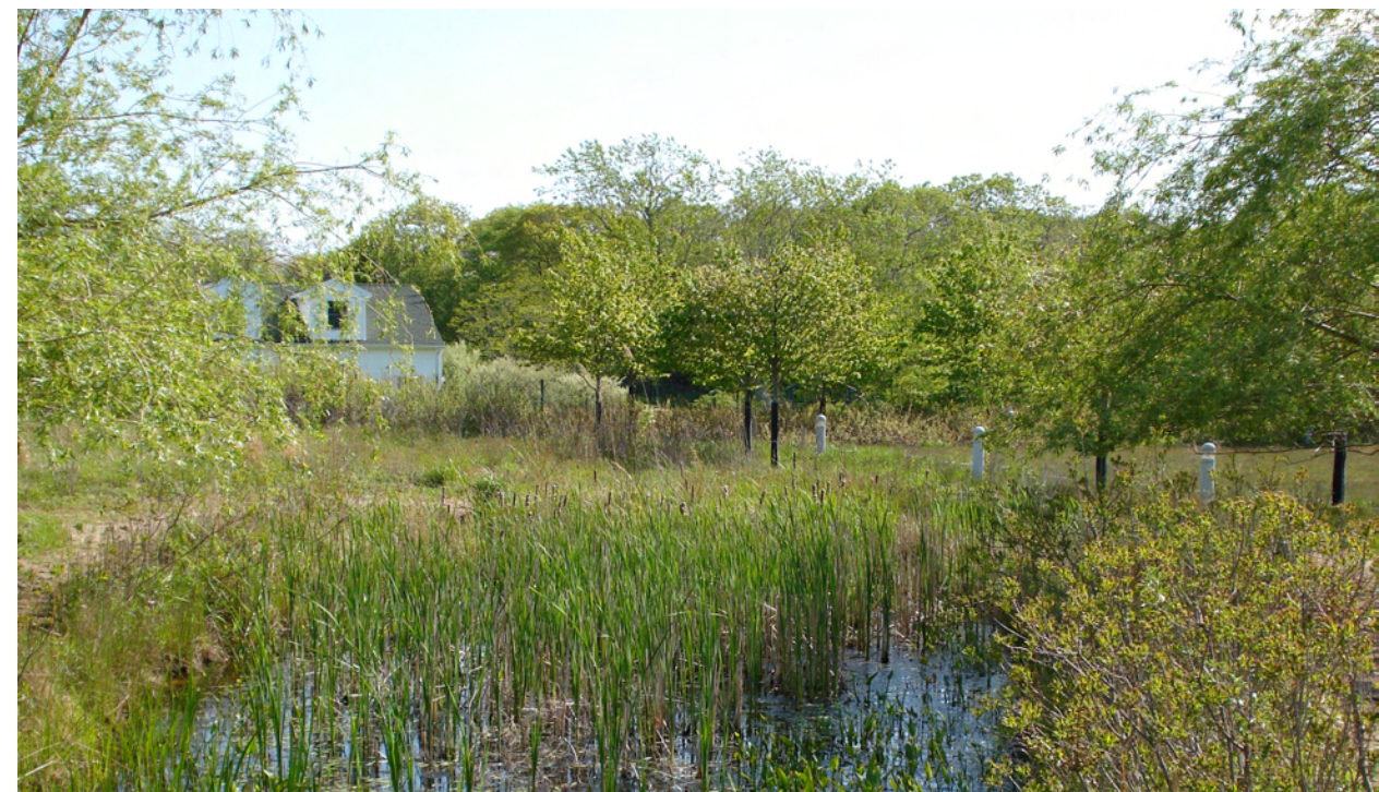
Constructed wetland restores the health to water body and provides cleansing of runoff from surrounding paved areas
