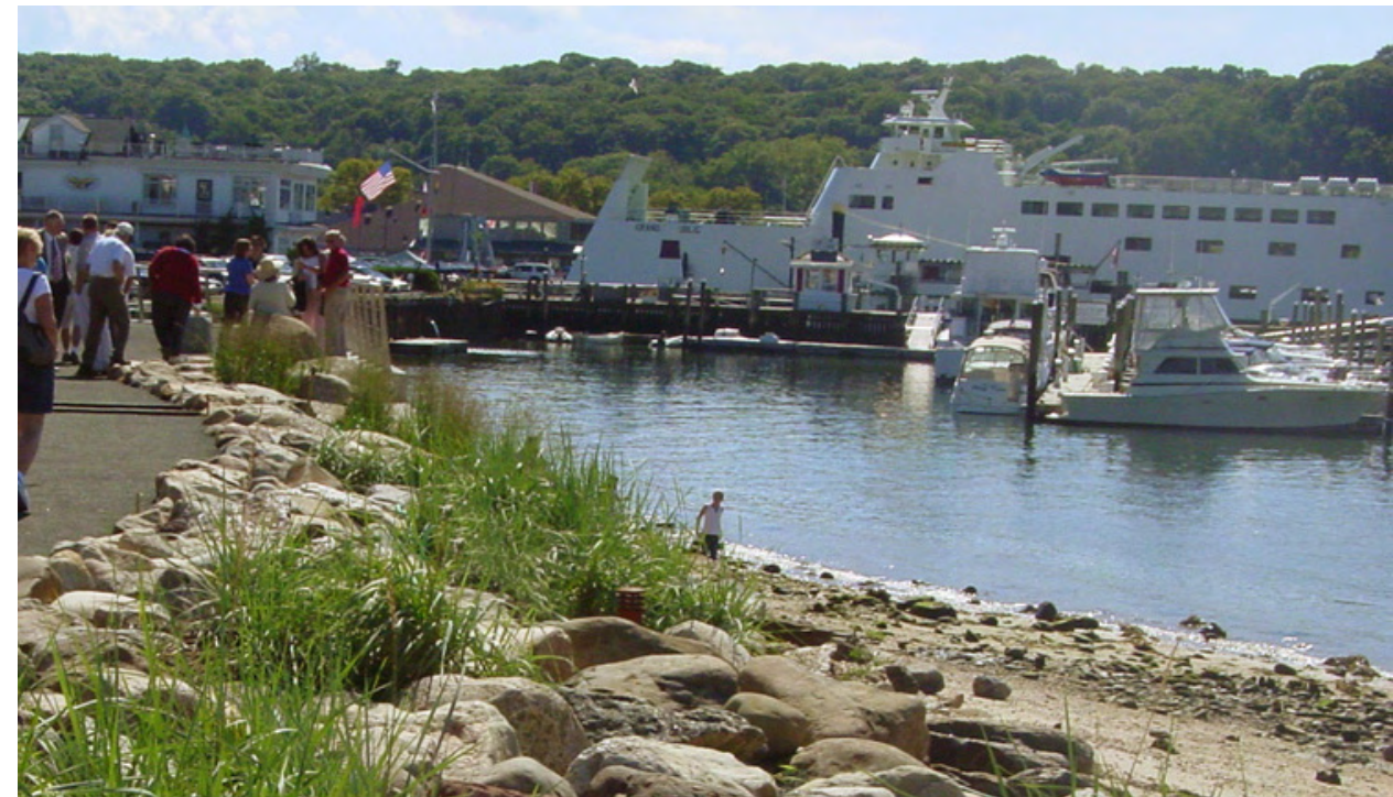
Natural rip-rap edging and planting protects and enhances shoreline
