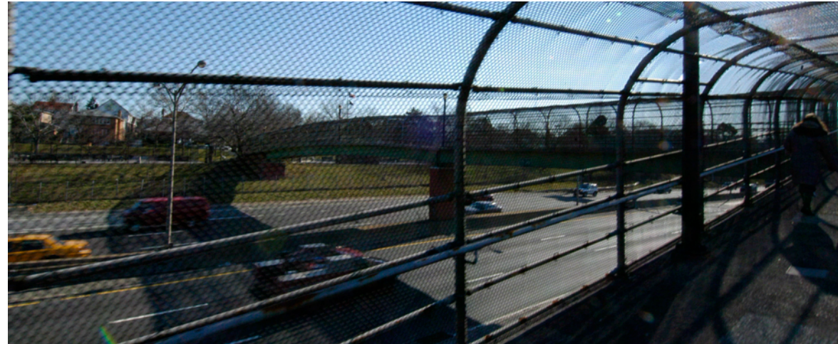
Pedestrian Bridge across the Van Wyck
