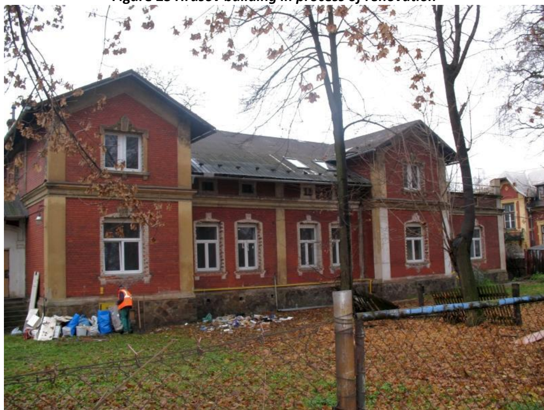
Figure 23 Hrušov building in process of renovation
