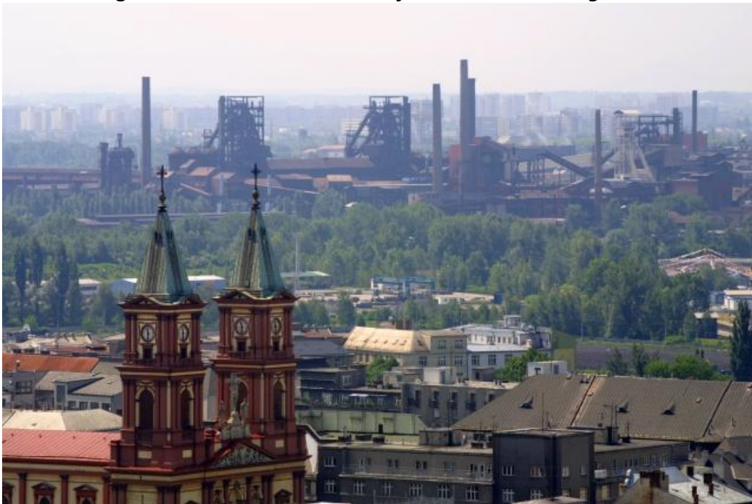
Figure 29 Lower Vítkovice blast furnaces in the background
