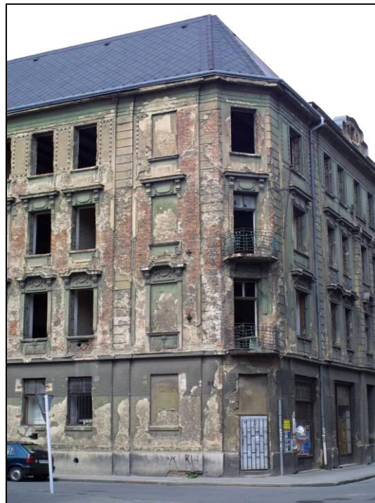
Figure 13 Building on Stodolní Street before reconstruction
