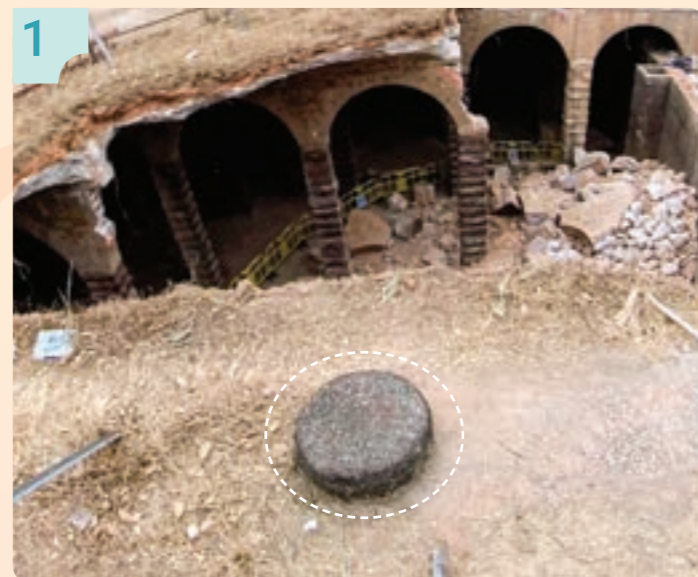
已封閉的通風井 Sealed Ventilator
