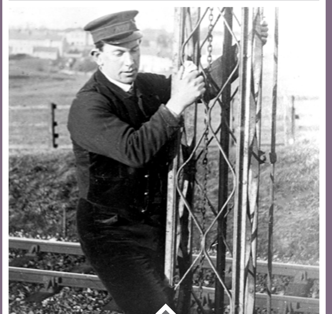
Railwayman climbing a signal. The chain for raising and lowering the oil lamp for filling and trimming is clearly visible, but the windlass for turning the mechanism would be at the bottom of the signal and is out of sight.
