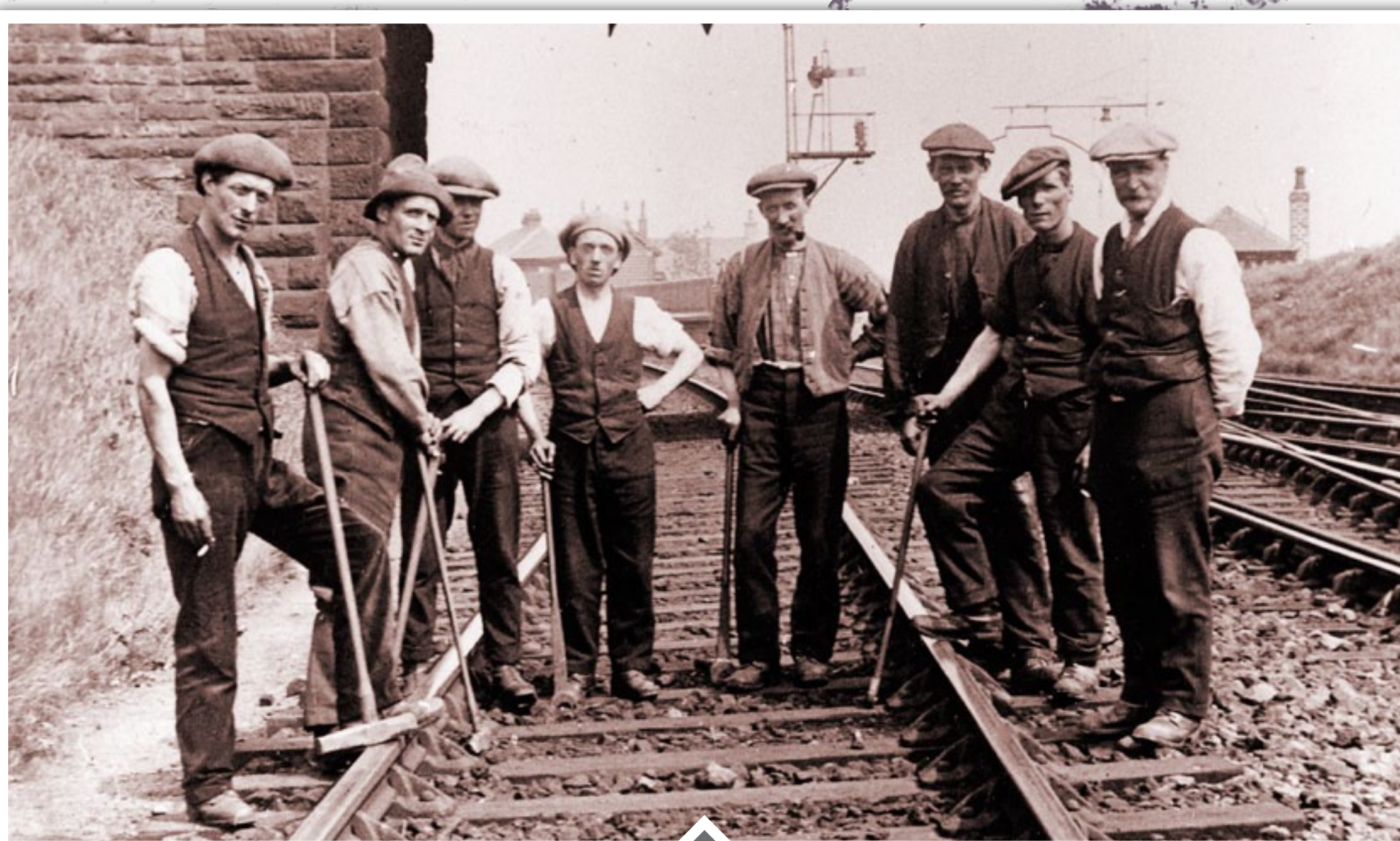
These surfacemen checked the railway lines and tracks around Blackridge
