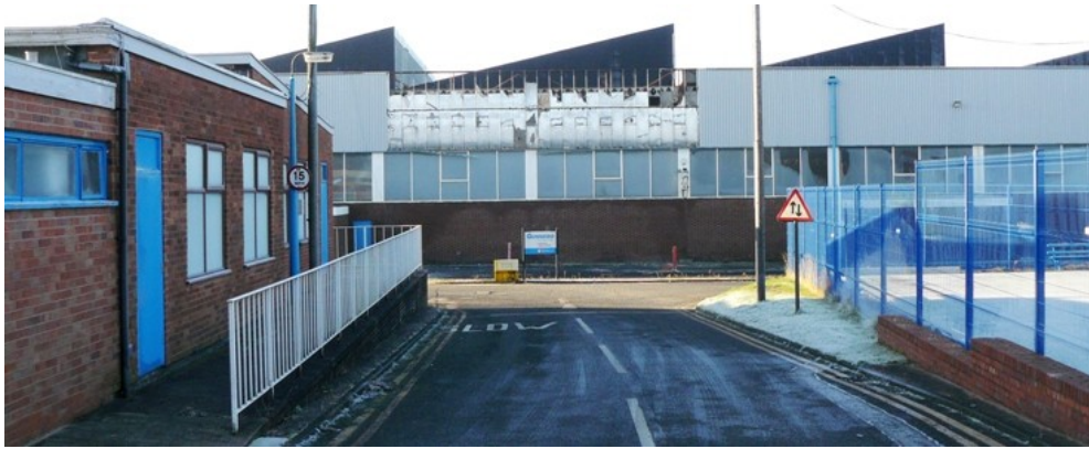
Figure 90 The former Chubb site to the east of Woden Road
