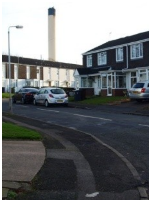
Figure 56 The cul-de-sac of Bramerton Close. A chimney on the site of New Cross Hospital is visible in the background (Photo D & L Cope)
