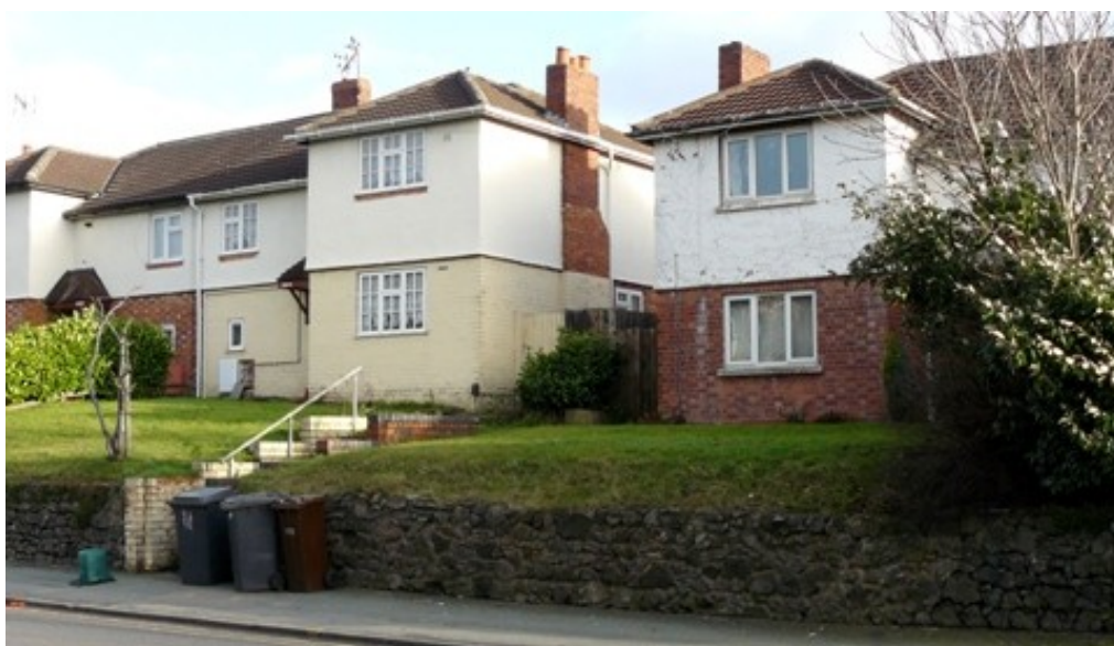
Figure 53 Interwar housing on the south side of Cannock Road. A long locally-distinctive clinker retaining wall fronts the properties (Photo: D & L Cope)
