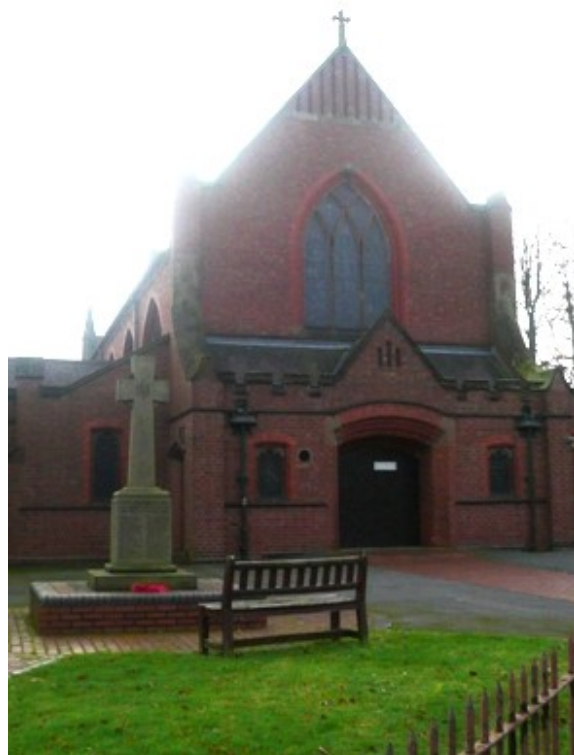
Figure 83 St Stephens Church (Photo: H Guest)
