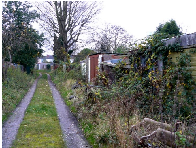
Figure 65 The southern end of the track showing garages at the
