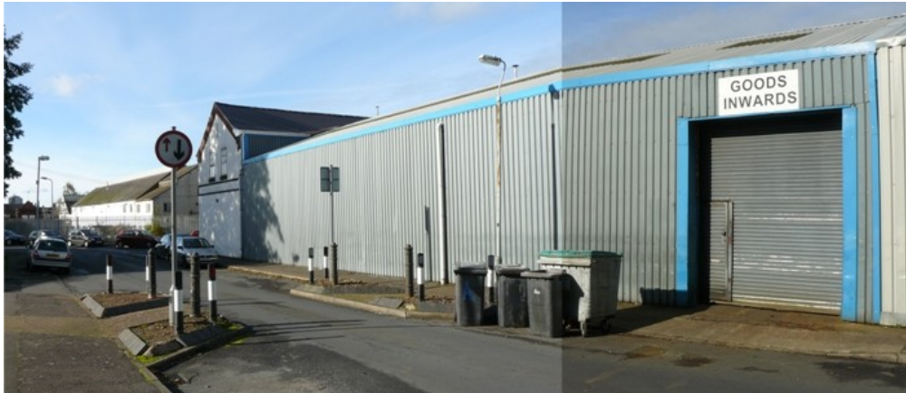
Figure 99 The original brick wall of this industrial building on Hobgate Road has been clad in corrugated steel since the aerial photograph was taken of it in 1992 (see above)
