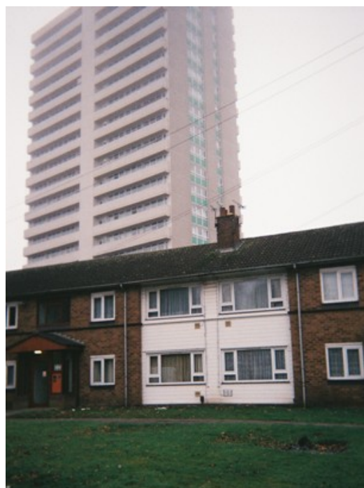
Figure 21 Grove Street with Longfield House at the rear (Photo D Williams-Smith)
