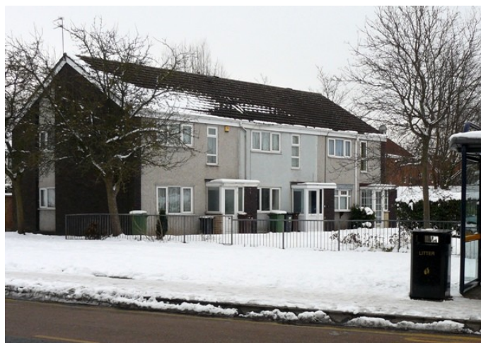
Figure 78 Housing on the north side of the Wyrley & Essington Canal
