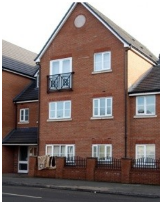
Figure 50 In the twenty-first century flats replaced a former dairy on Prestwood Road (Photo: D & L Cope)
