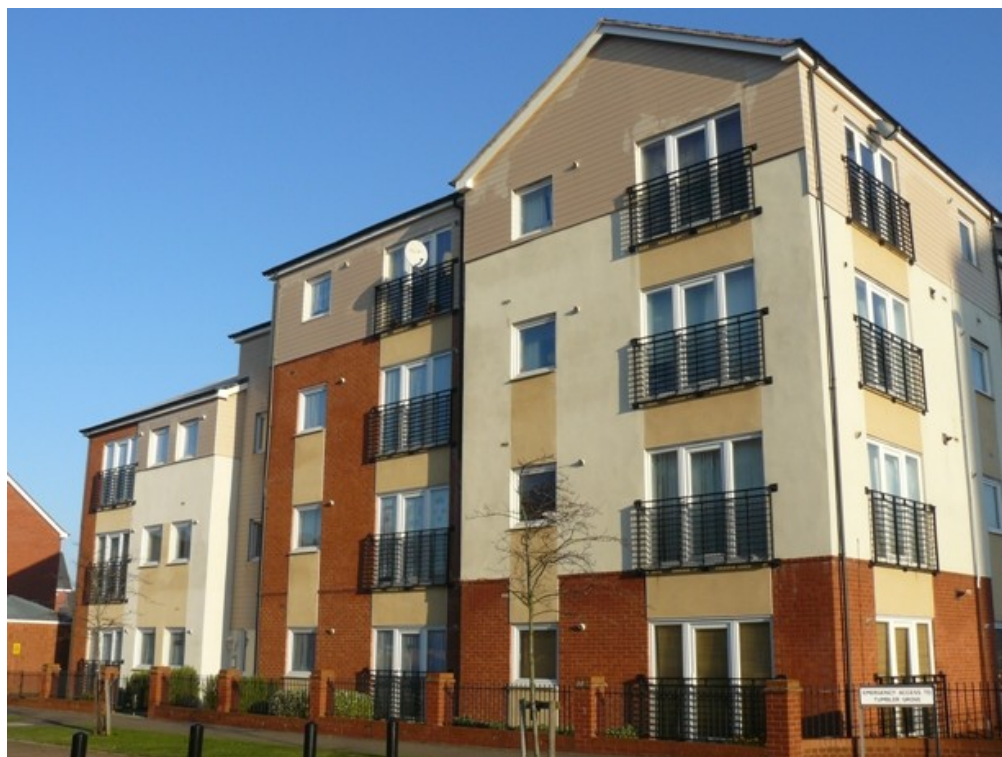
Figure 102 Four storey flats on the corner of Wednesfield Road and Tumbler Grove
