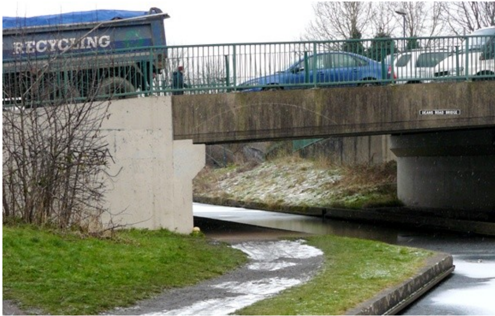
Figure 79 The Dean's Road Bridge over the Wyrley & Essington Canal
