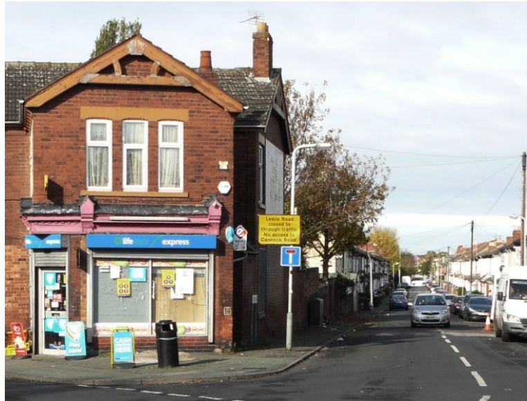
Figure 60 The shop at the corner of Powell Street and Leslie Road
