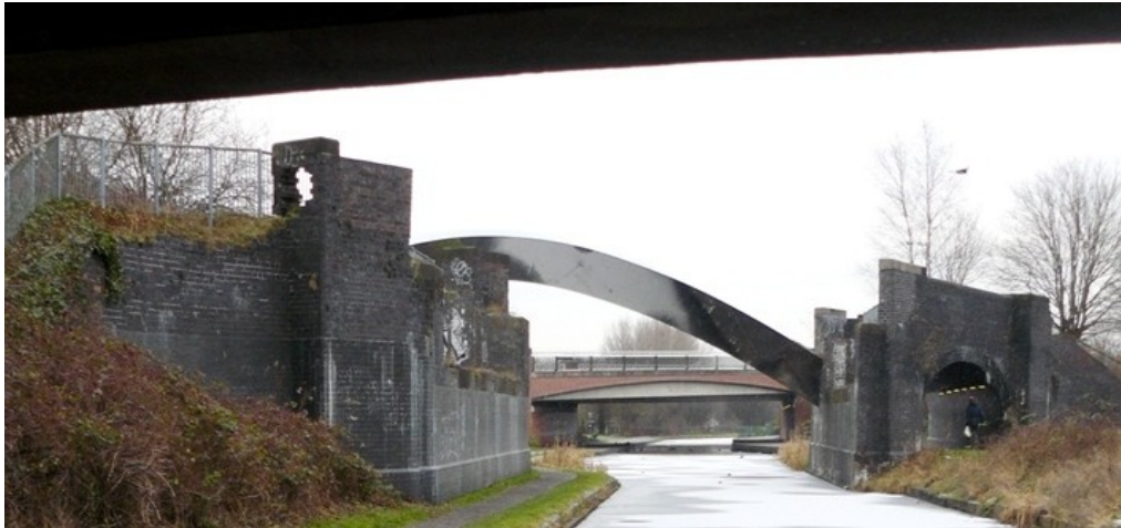
Figure 72 The remains of a 19th century railway bridge over the Wyrley & Essington canal is now the location of an elegant piece of public art which provides a reminder of the crossing. What's left of the old structure is seen here between two twentieth century road bridges (carrying Dean's Road and Wednesfield Way)
