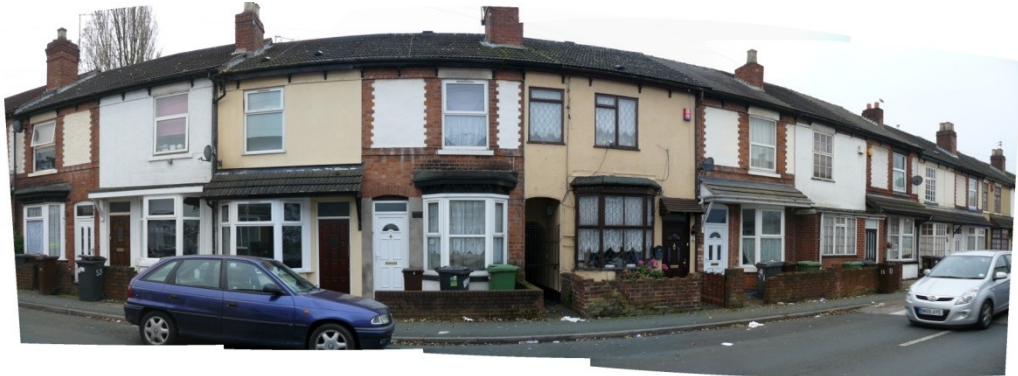
Figure 63 The narrow tunnel-back terraced houses on the west side of Leslie Road
