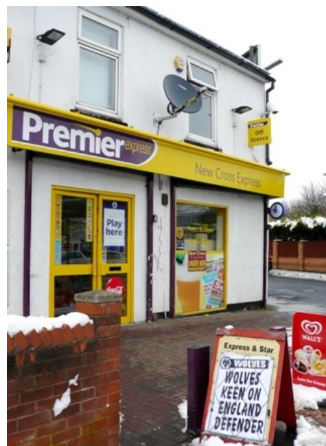
Figure 14 The shop at the corner of Coronation Road and Wolverhampton Road
