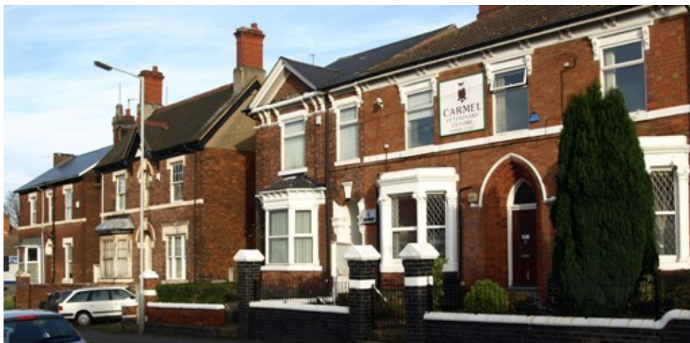
Figure 51 Bushbury road between Milton Road and Thorneycroft Lane (Photo: D & L Cope)
