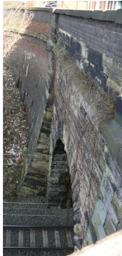
Figure 74 The northern end of Heath Town Tunnel
