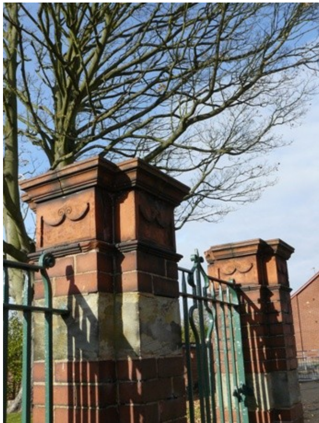
Figure 100 Gate piers outside St Stephen's school, Woden Road
