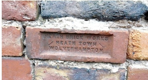
Figure 37 Local bricks used here as part of a twentieth century wall separating the site of Heath Park School and the former 'North Farm' on Prestwood Road. The production of bricks, tile, and terracotta has been a significant local industry.
