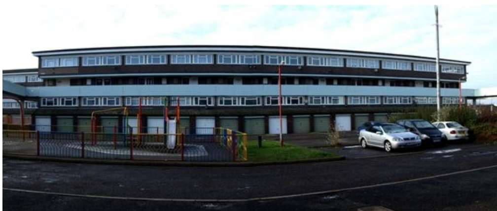
Figure 42 One of eight blocks of maisonettes within the development (Photo: D & L Cope)
