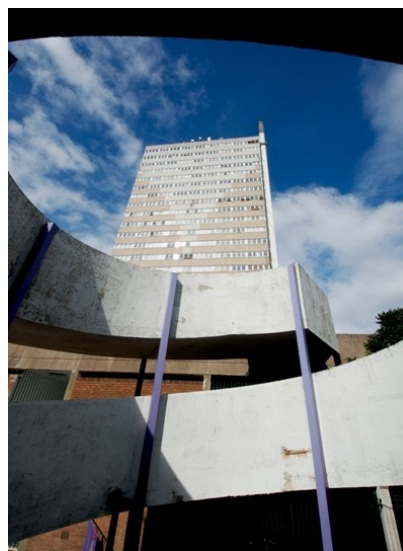
Figure 23 The ramp to Heath Town Estate on Wednesfield Road (Photo: Matthew Whitehouse)
