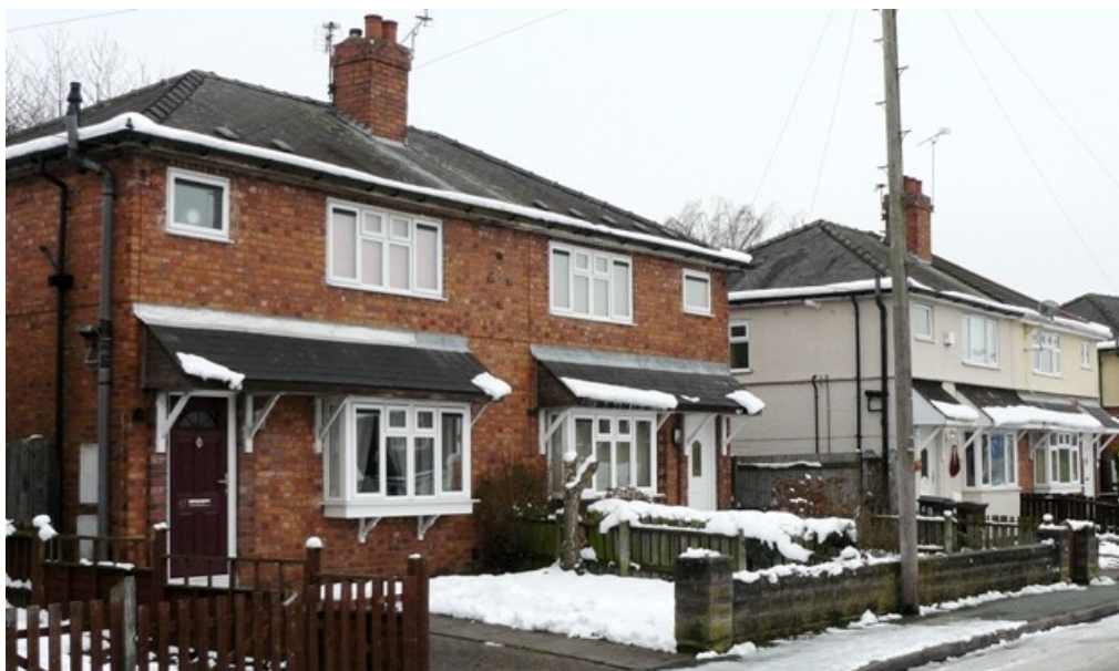
Figure 9 Semi-detached interwar properties on Coronation Road
